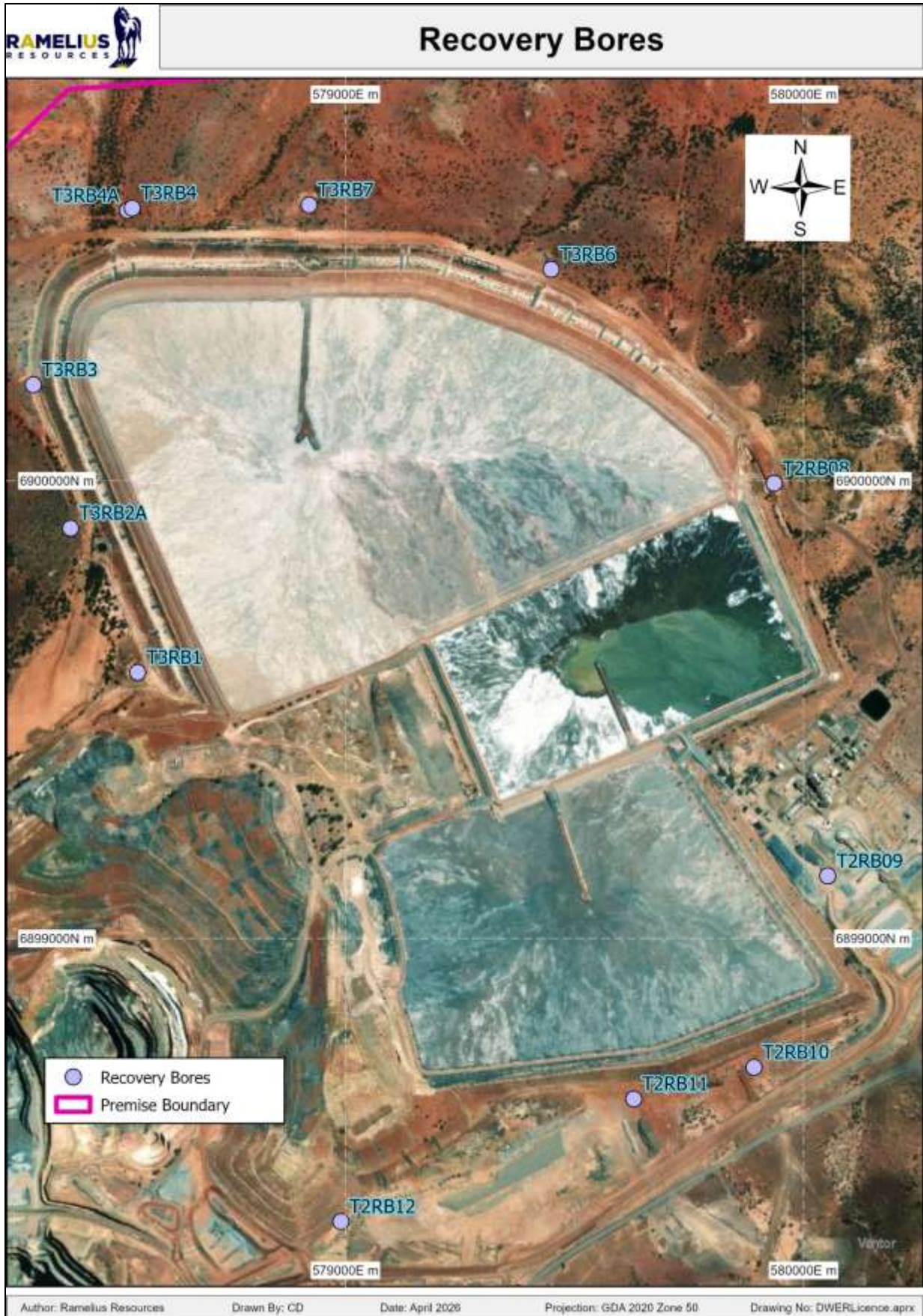
Figure 3: seepage recovery bore locations
