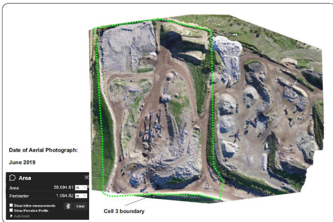
Figure 2: Proposed designated Asbestos Disposal Area (“Cell 3”), located on the western portion of Lot 434.
