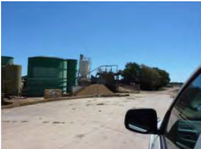
Photo 8 – WWTP showing separated solids within bunded area
