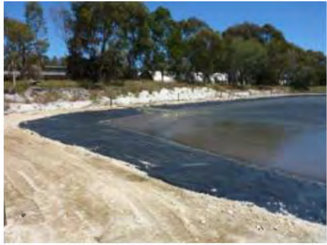
Photo 10 – Pond 0 inlet from WWTP
