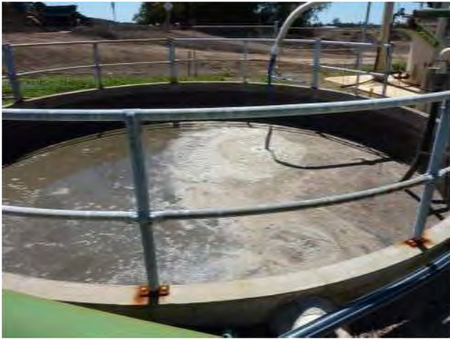
Photo 9 – WWTP discharge pit
