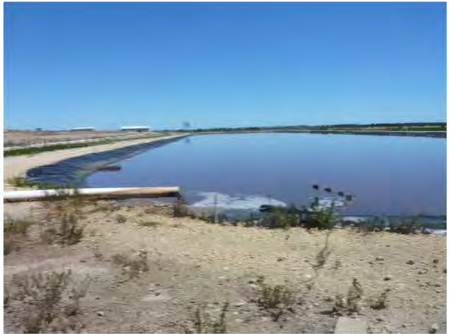
Photo 12 – Pond 2 inlet from Pond 0
