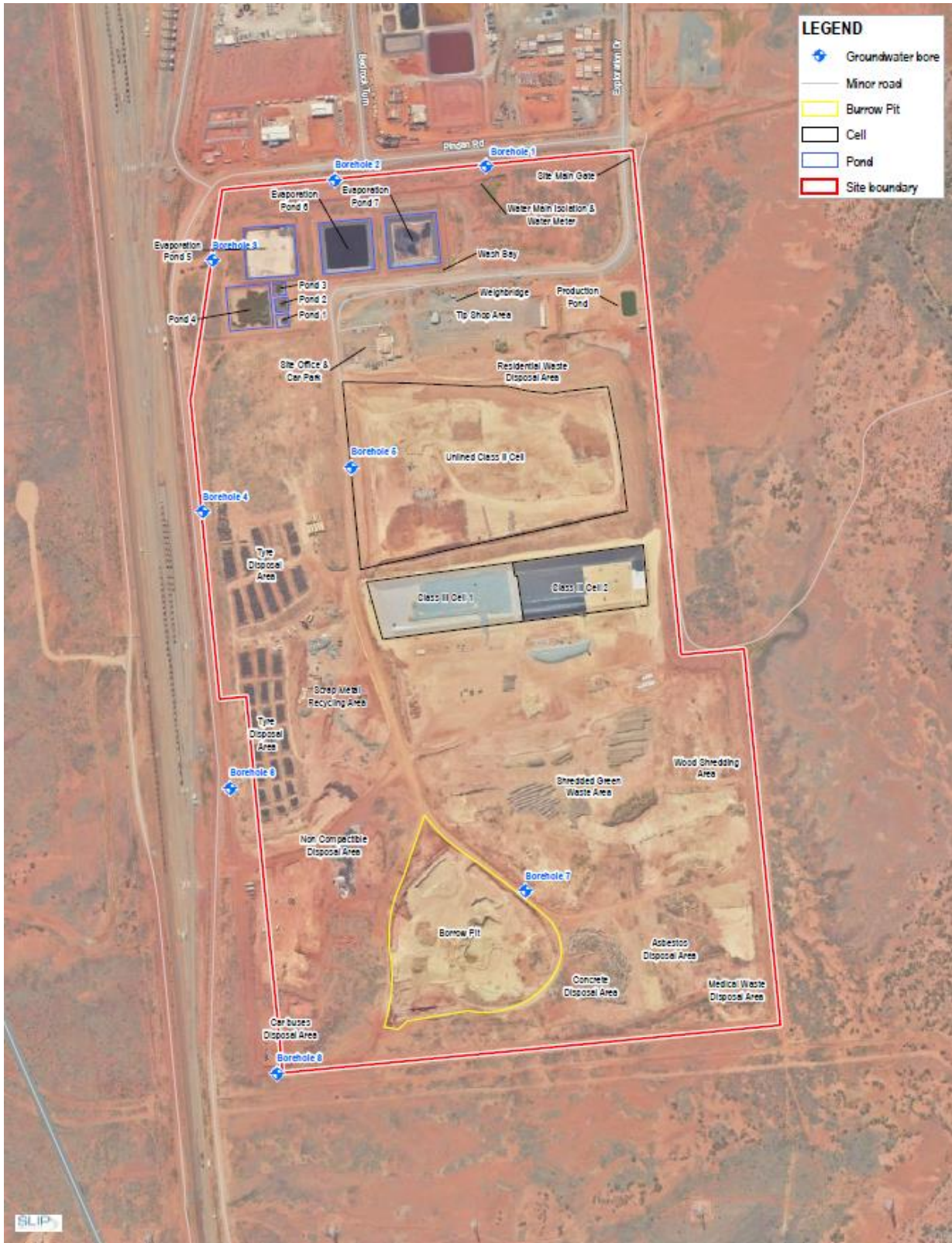
Figure 1: Aerial overview of Premises
