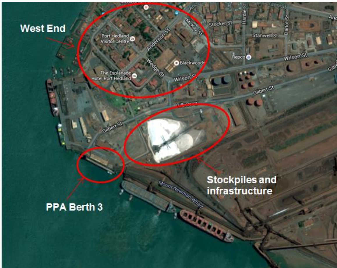
Figure 2 - Aerial image of the location of the Premises in comparison to the West End
