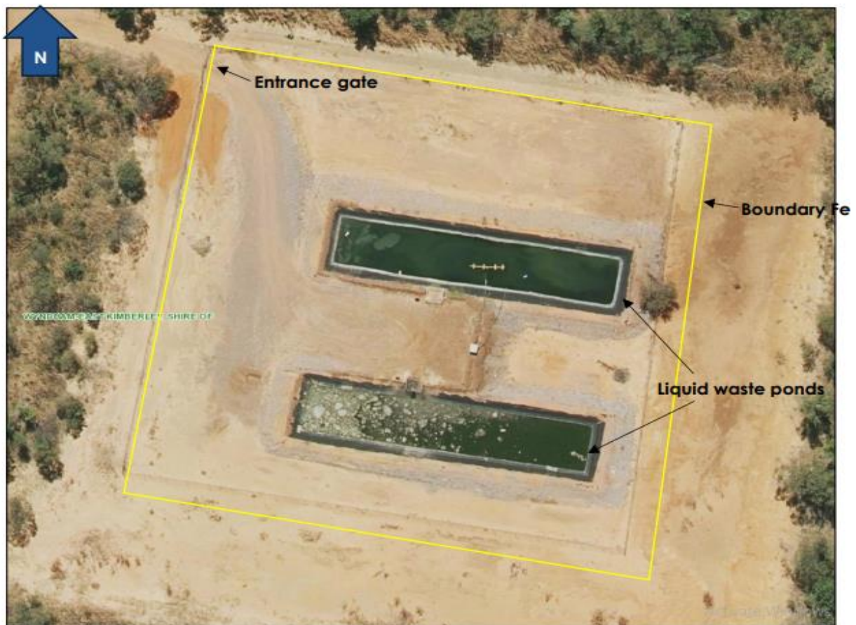
Figure 1: Liquid waste ponds
