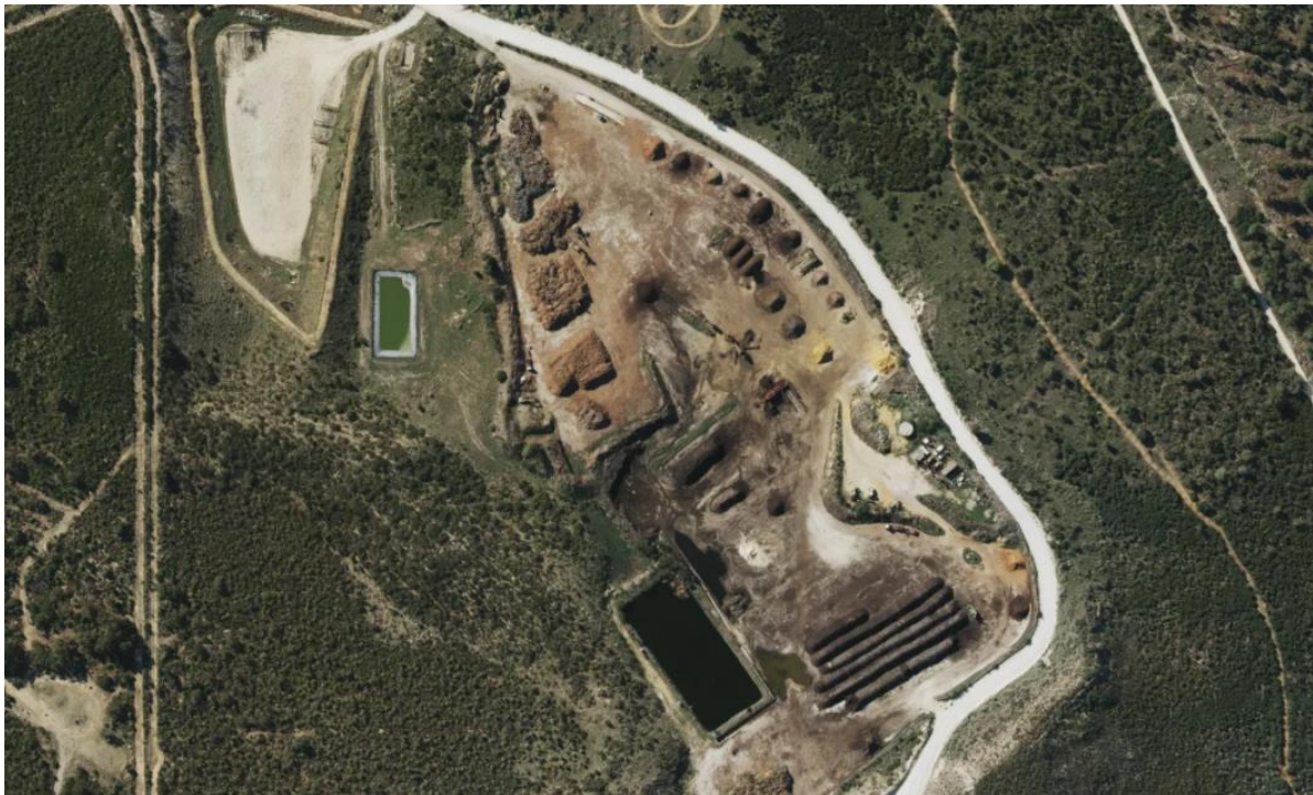
Figure 1 Aerial imagery – 23 April 2023 (Source: MetroMap)
