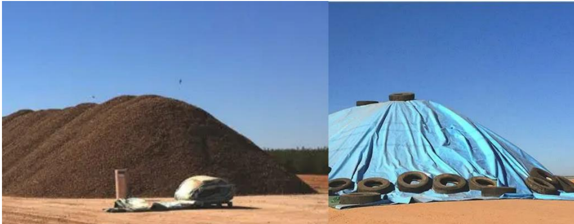
Figure 5 Example of tarpaulin temporary stockpile cover
