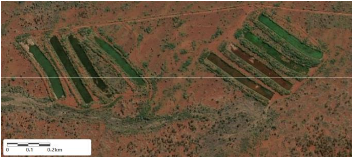
Figure 1: Packsaddle Infiltration Ponds
