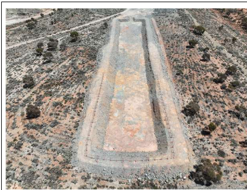
Figure 2: Photo of completed landfill cell taken from Environmental Compliance Report (APP-0032200).
