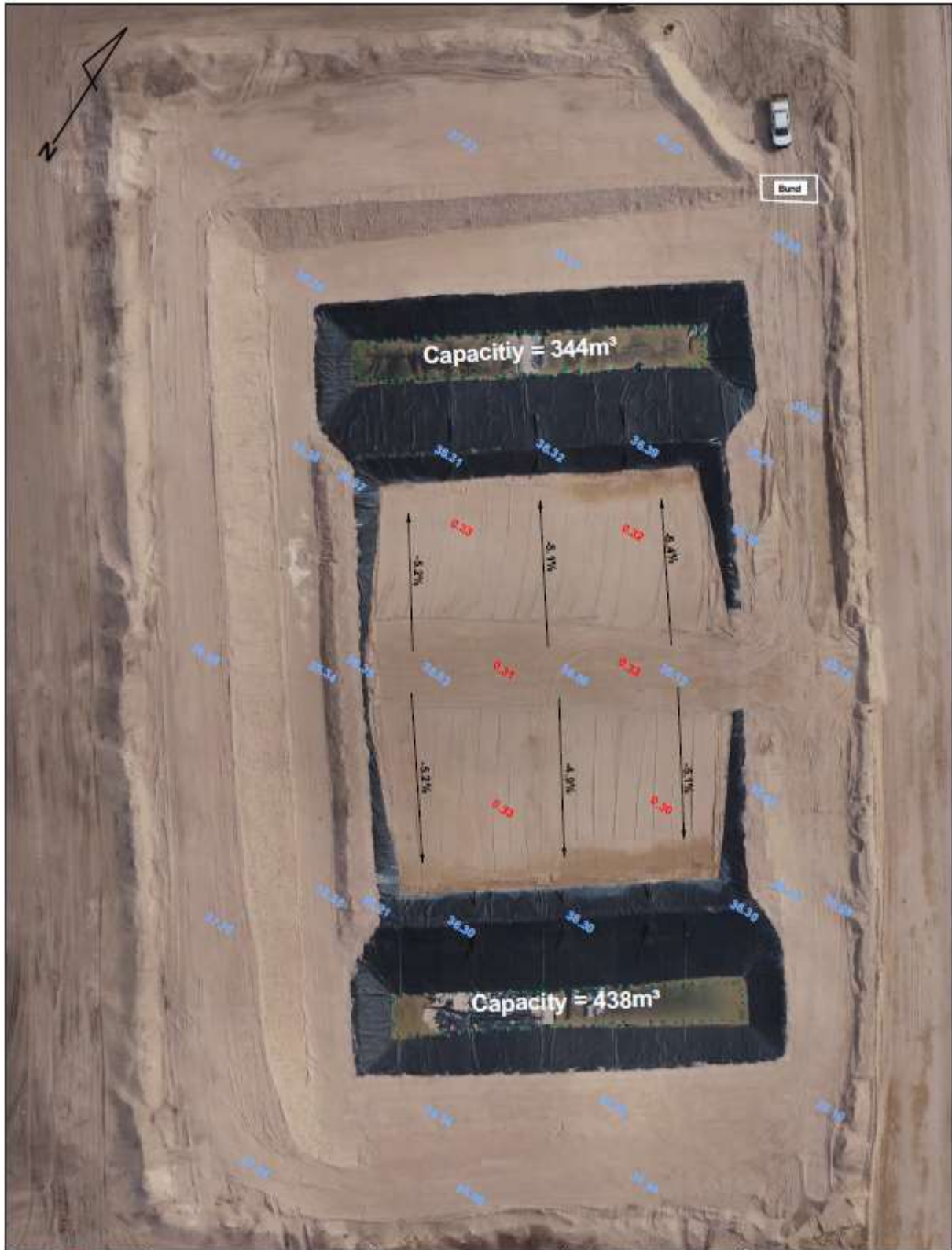
Figure 1: Completed Bioremediation facility
