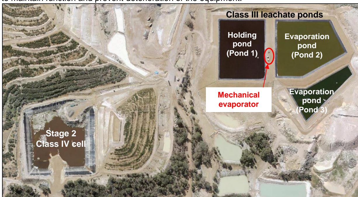
Figure 2: Stage 2 Class IV cell and Class III leachate ponds (aerial imagery August 2019).
