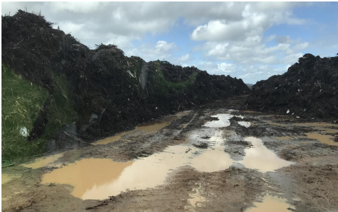
Figure 7: Stormwater/leachate pooling on the green waste processing hardstand, September 2019
