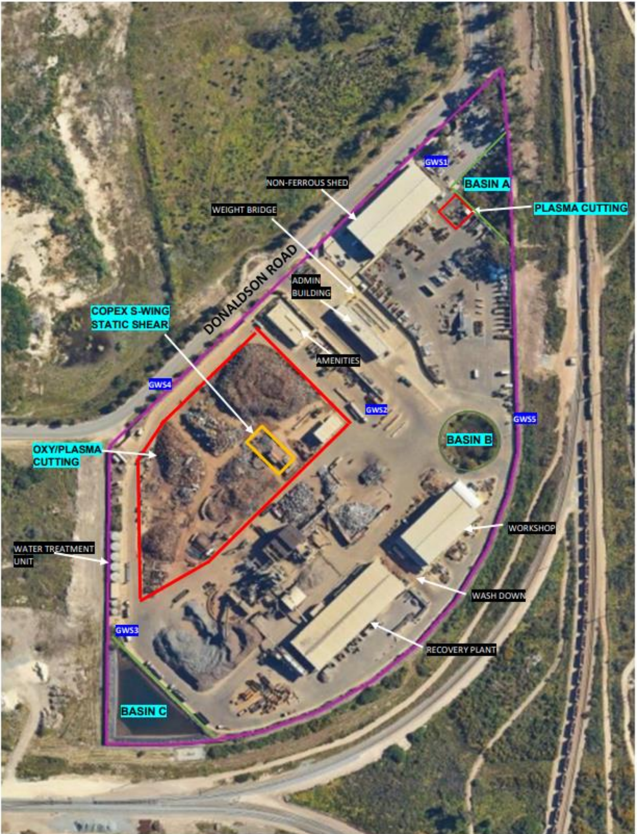
Figure 1: Location of Shear and Oxy/Plasma cutting on the premises
