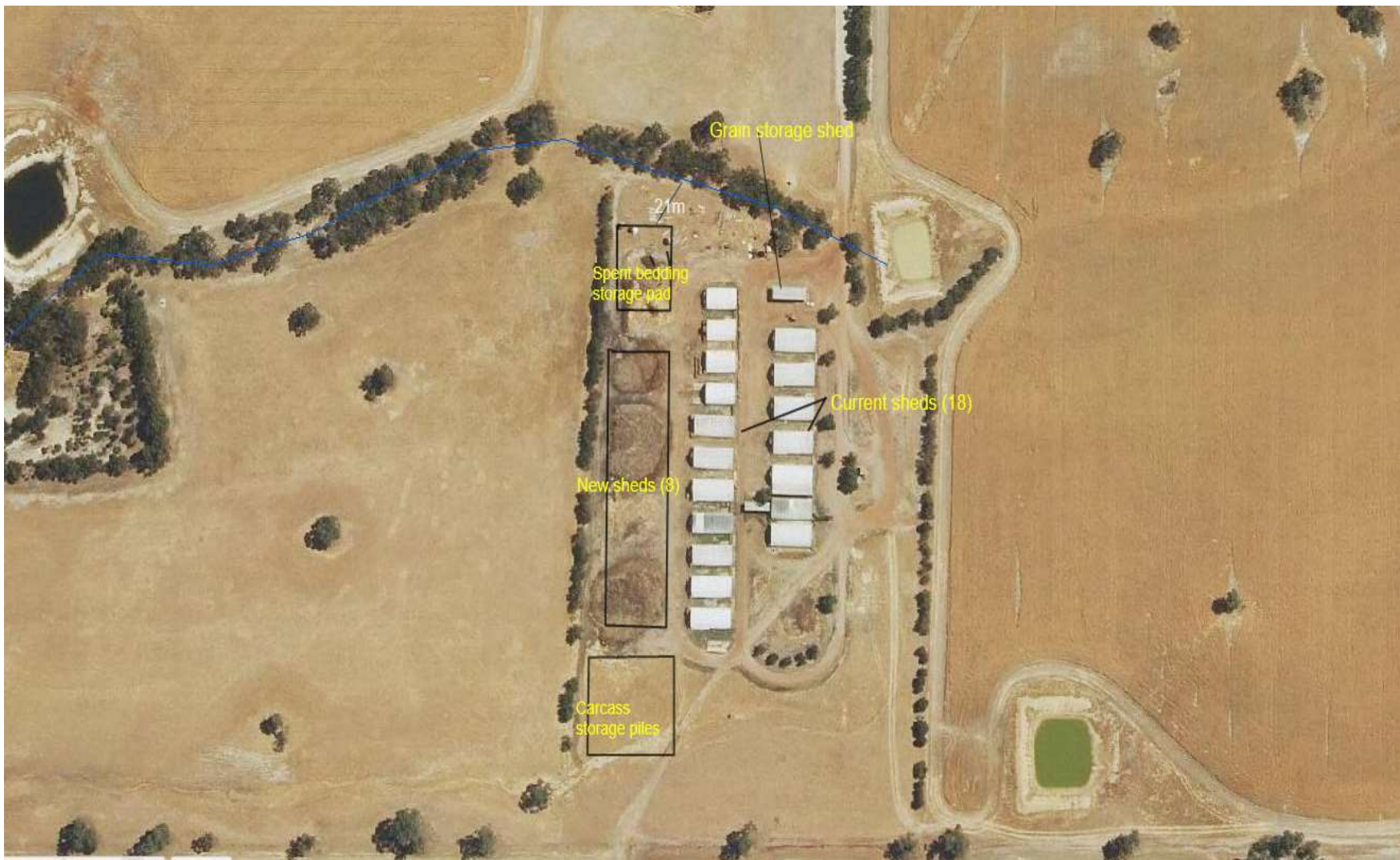
Figure 4: Infrastructure at Adelong Farm (DWER generated)
