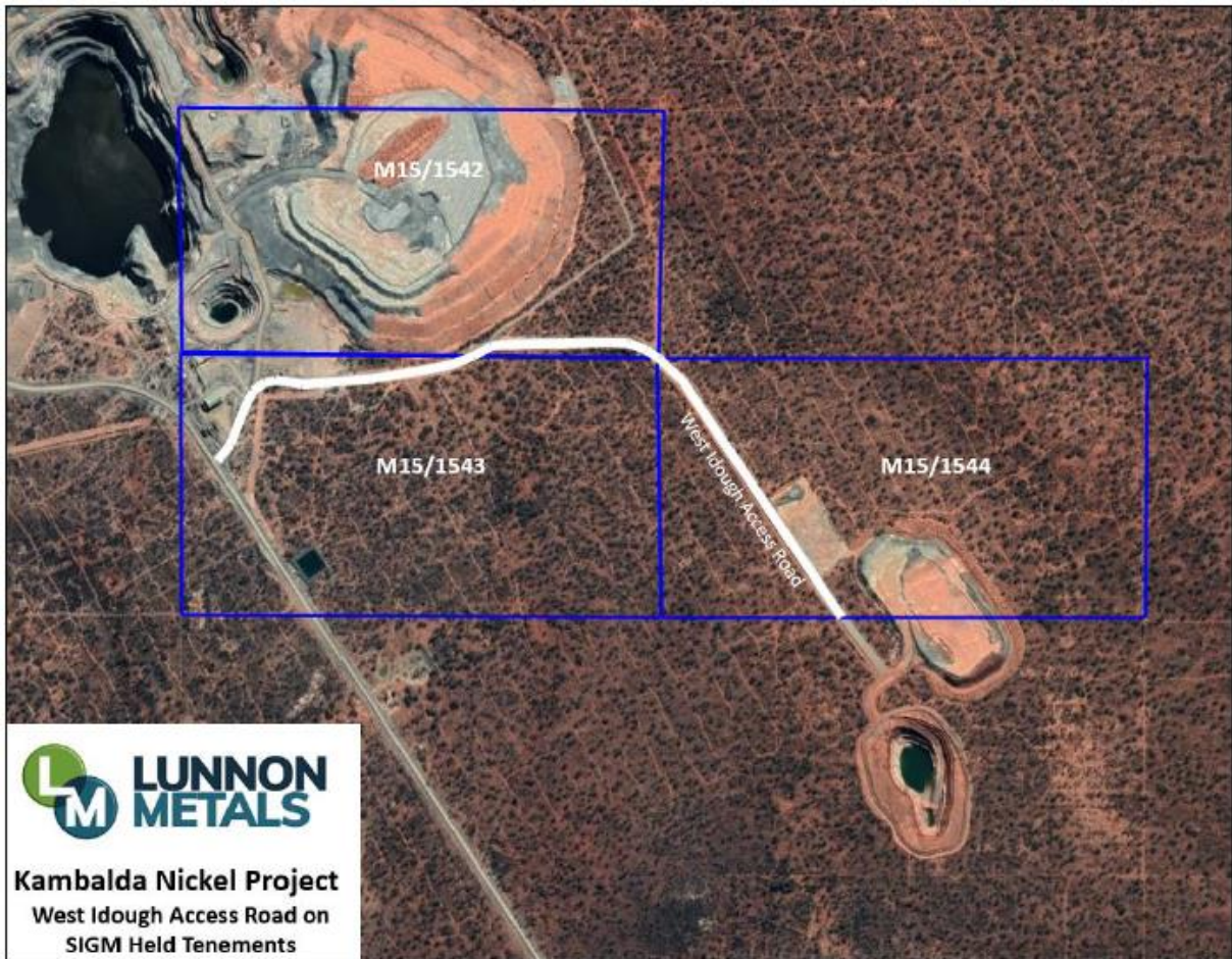
Figure 3: West Idough Haul Road/Baker Road access
