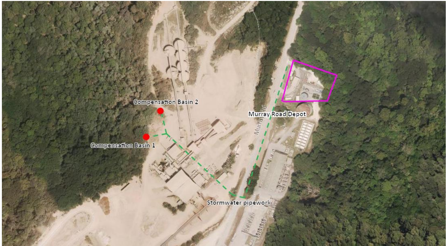
Figure 1: Current stormwater pathway from the Murray Road Depot to Compensation Basins 1 and 2
