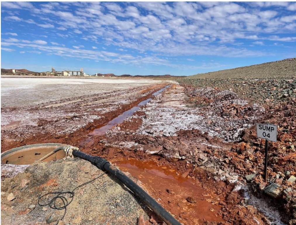
Figure 6: Interception trench and sump (SP4) (Sourced from GRM 2024)
