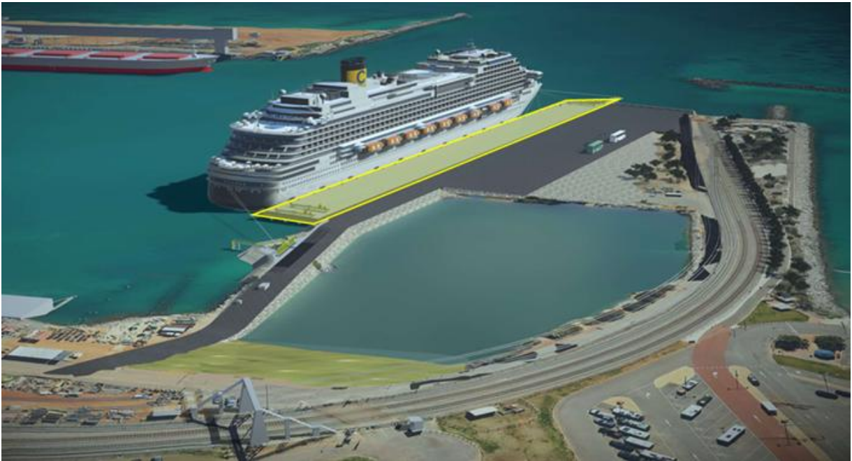
Figure 2: Berth 1 render new wharf highlighted yellow
