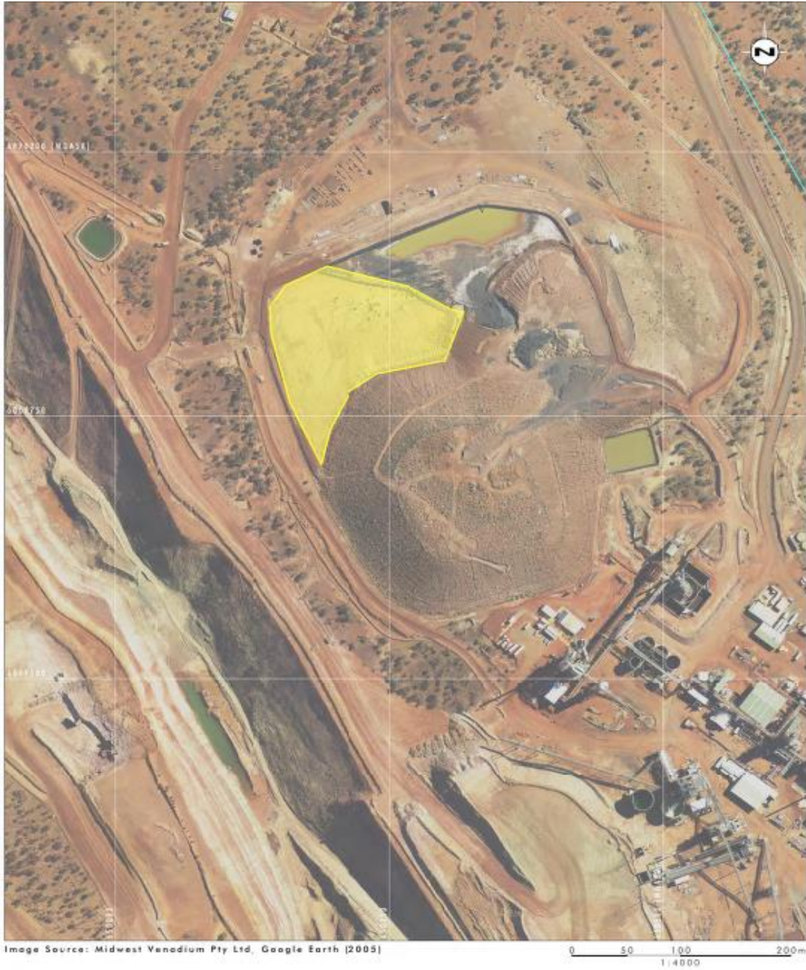
Figure 6: Aerial view of the CTSF showing the extension area in yellow planned for GCL and HDPE liner installation (Umwelt, November 2019)
