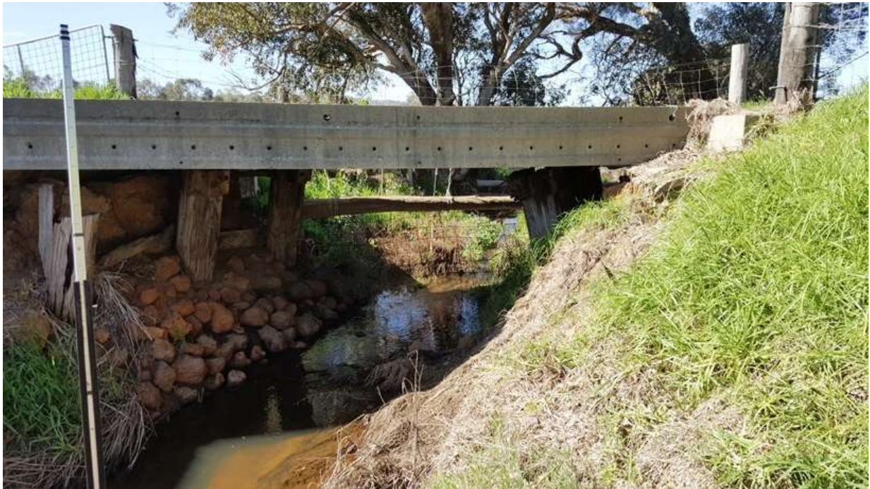
Figure 4. Drakesbrook drain adjacent to Premises
