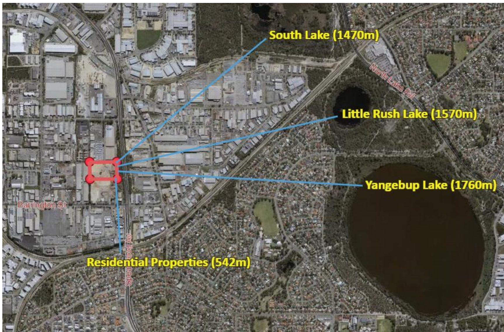
Figure 3: Distance to receptors - the Premises boundary is defined by the red line.
