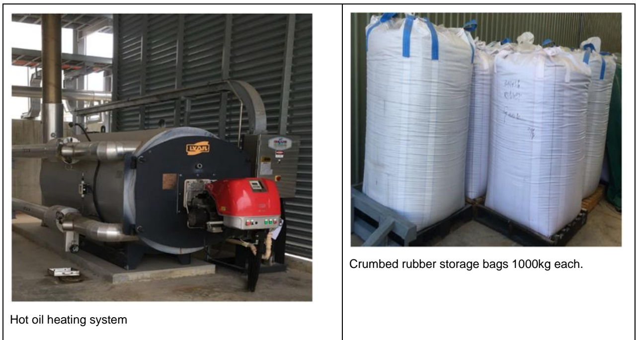
Figure 4: Hot oil heating unit and crumbed rubber storage bags
