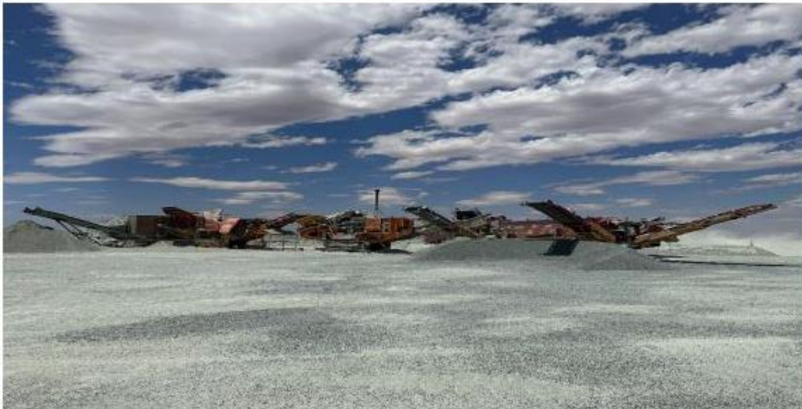
Figure 2: Showing Crushing and Screening Plant in Situ
