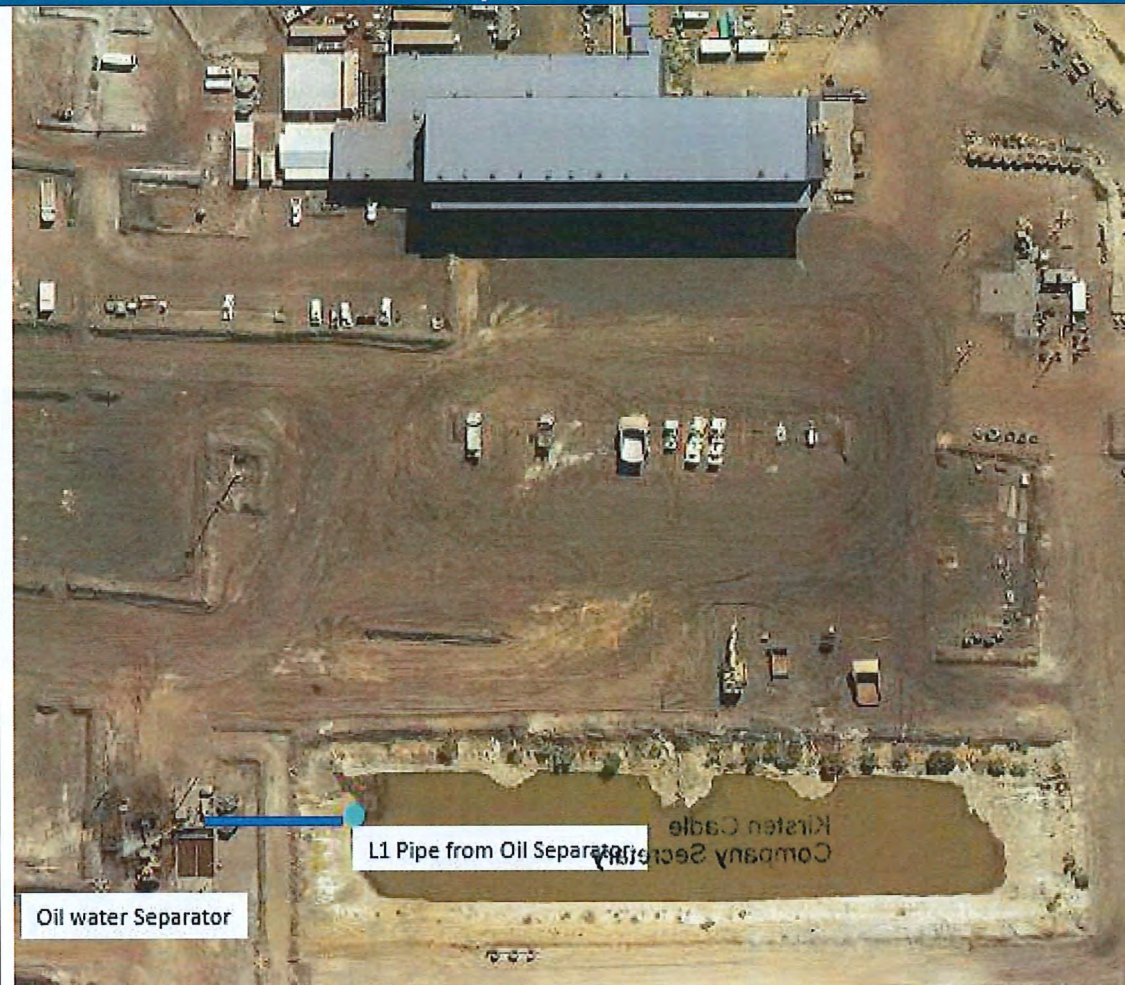
Figure 3: Location of L1 discharge point for treated water from the Oil Water Separator.
