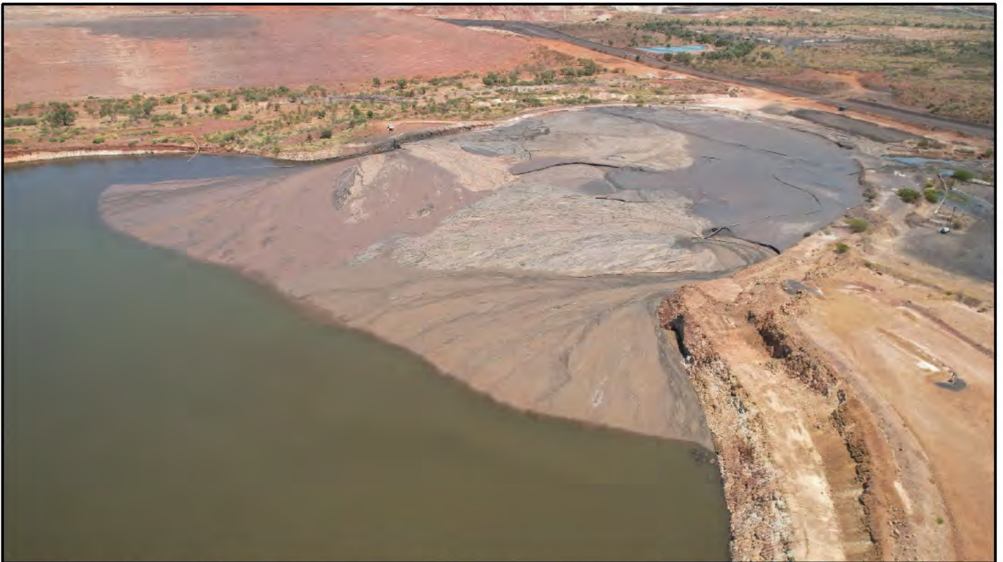
Photo 02: HSPTSF (active) northern discharge location and tailings beach, looking southwest.
