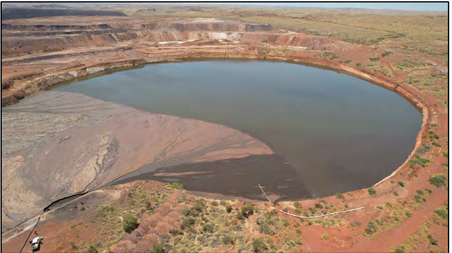
Photo 06: HSPTSF (active) supernatant pond, from southern discharge location, looking northeast.
