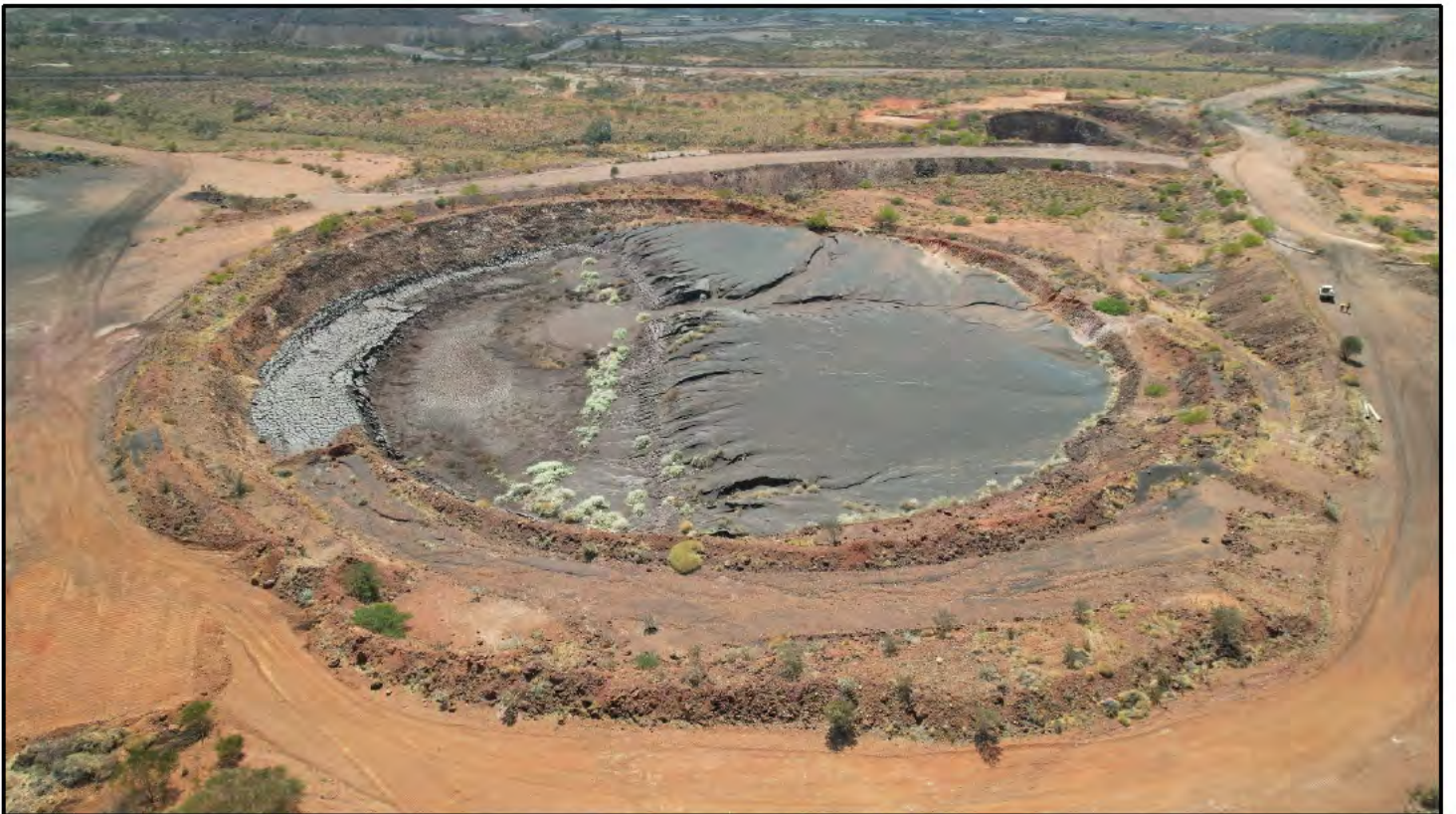
Photo 24: View of Dartmoor Pit – DaPTSF (in-active), looking east.
