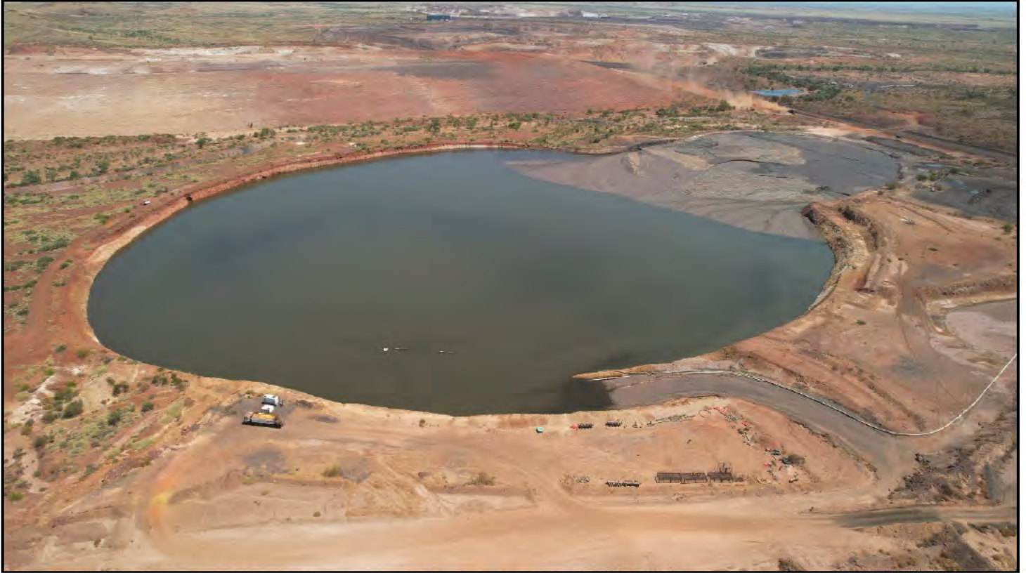
Photo 01: View of Homestead Pit - HSPTSF (active) from decant position, looking southwest.
