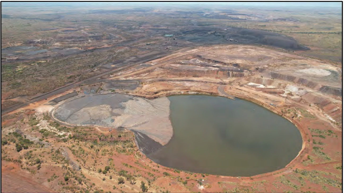
Photo 12: View of HSPTSF (active) from southeast perimeter, looking northwest.
