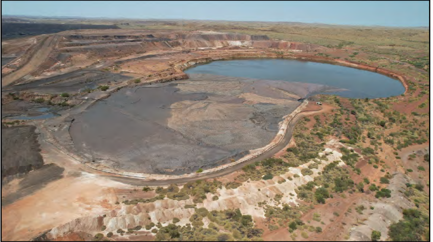
Photo 05: HSPTSF (active) tailings beach from southwest perimeter, looking northeast.
