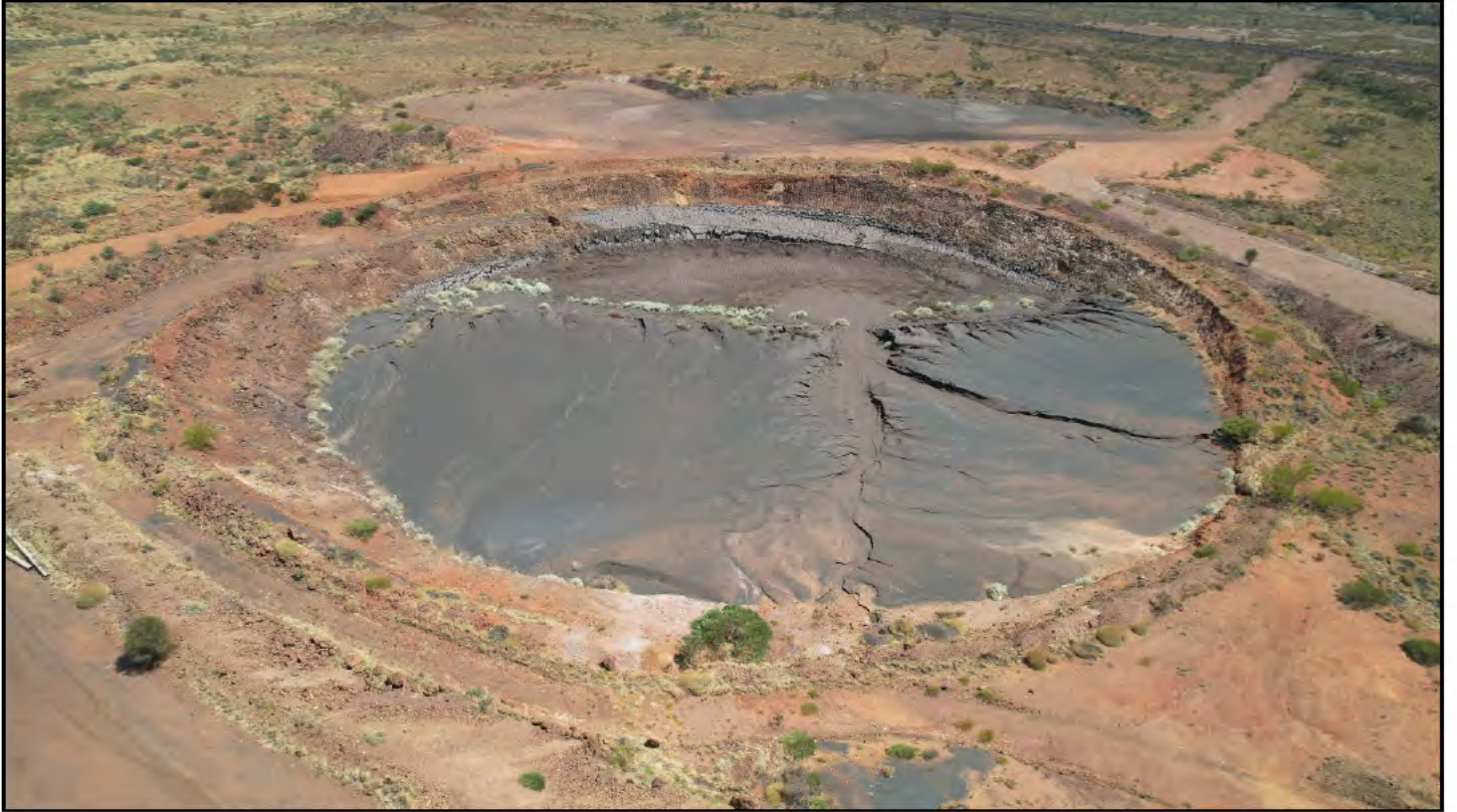
Photo 23: View of Dartmoor Pit – DaPTSF (in-active), looking north.
