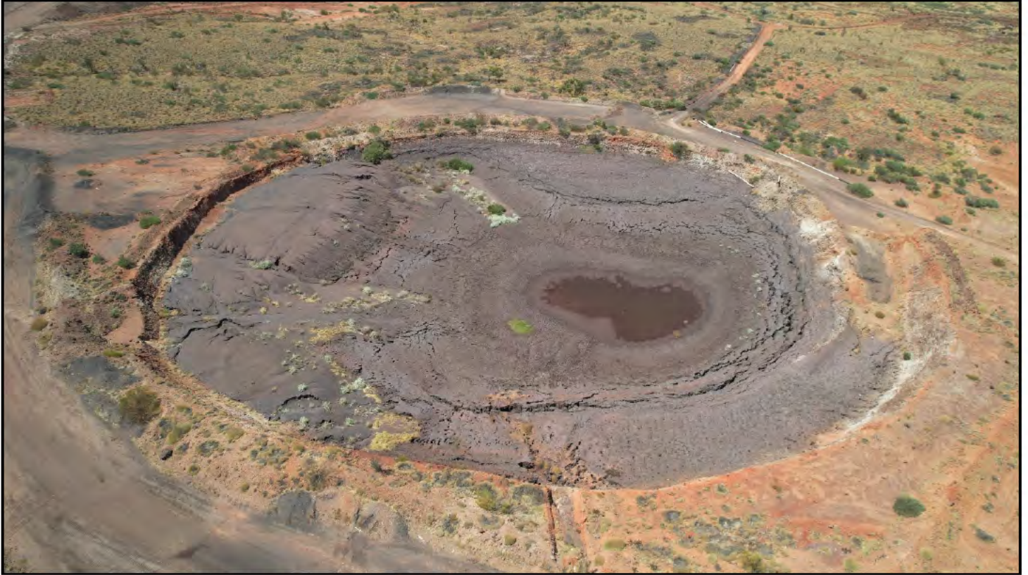
Photo 17: View of Malta Pit – MPTSF (in-active), looking south.
