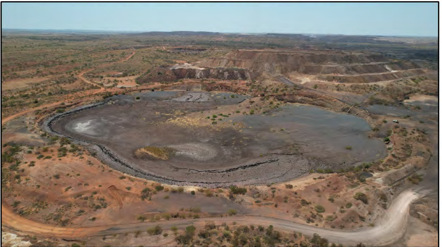
Photo 14: View of Area 1 Pit – A1PTSF (in-active), looking west.
