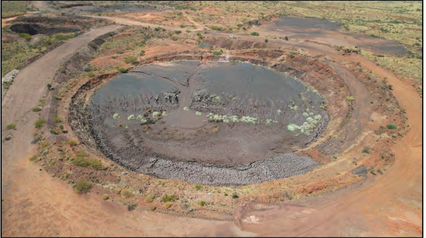
Photo 21: View of Dartmoor Pit – DaPTSF (in-active), looking south.
