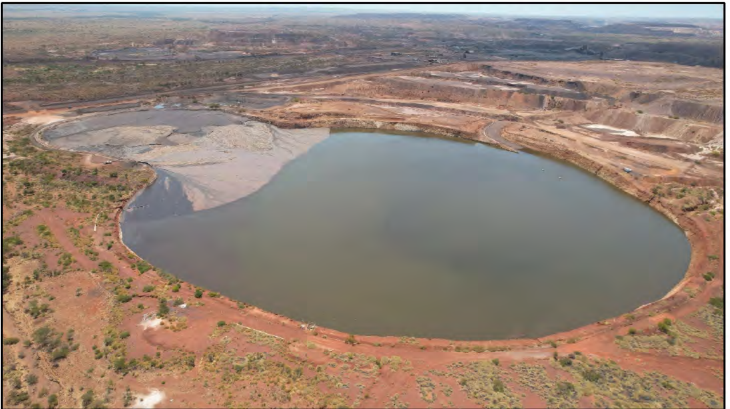
Photo 08: HSPTSF (active) from southeast perimeter, looking northwest.
