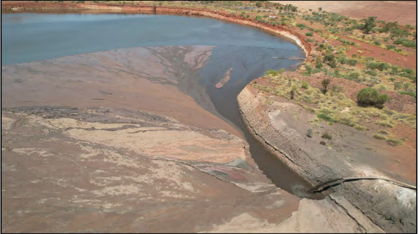
Photo 09: HSPTSF (active) tailings deposition from southern discharge location, looking southeast.
