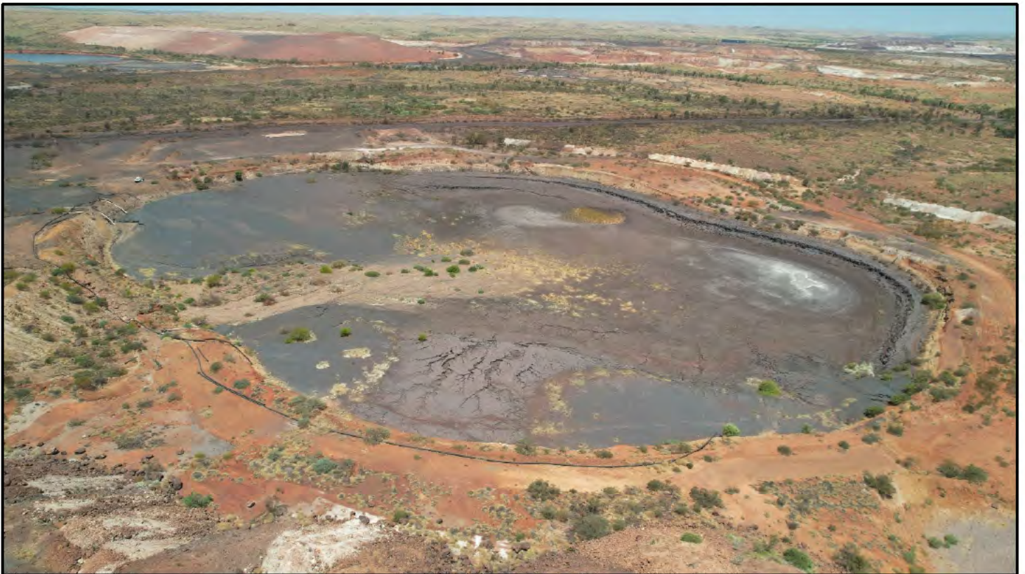
Photo 16: View of Area 1 Pit – A1PTSF (in-active), looking east.
