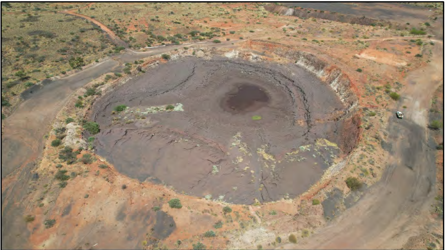
Photo 18: View of Malta Pit – MPTSF (in-active), looking west.
