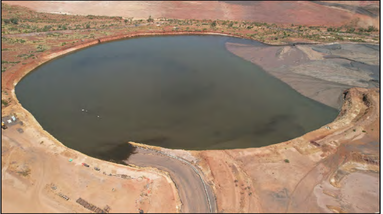
Photo 11: HSPTSF (active) decant location and supernatant pond, looking south.
