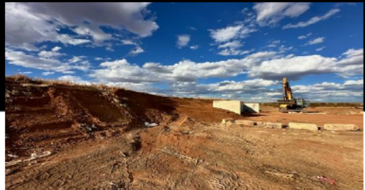
Photograph 7b: Clean fill to cover the excavated portion
