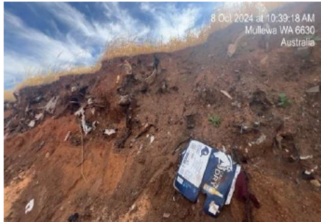
Photograph 9a: Exposed landfill section showing layers of mixed waste materials.
