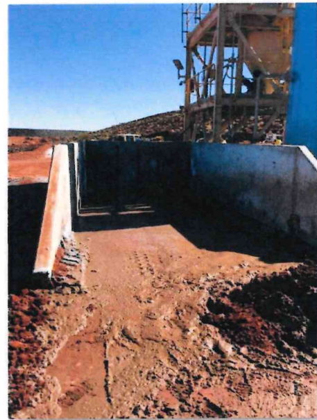
Figure 4- Sump discharge location
