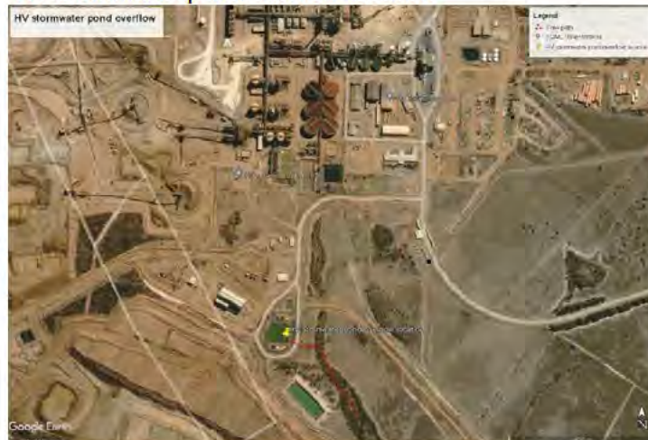
HV stormwater pond overflow location
