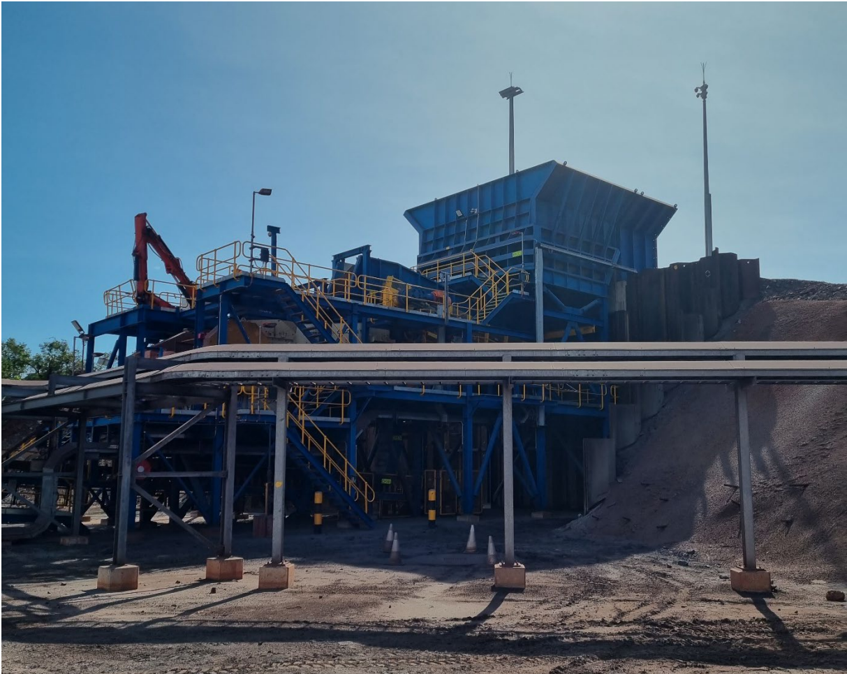
Figure 3: New primary crusher
