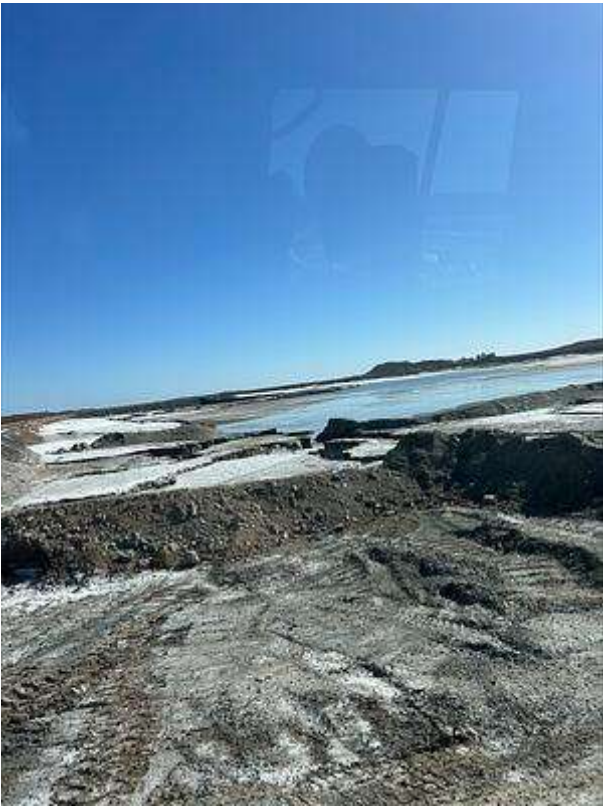
Upload photo from north-west corner toward centre decant well
