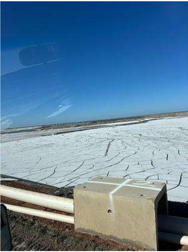
Upload photo from south-west corner toward centre decant well
