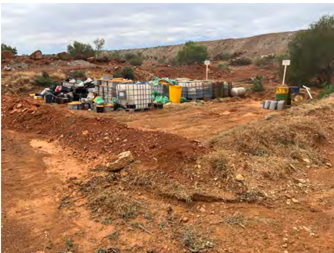
Figure 3-7: New windrow across hydrocarbon bund – excluding surface water (Feb 2026)
