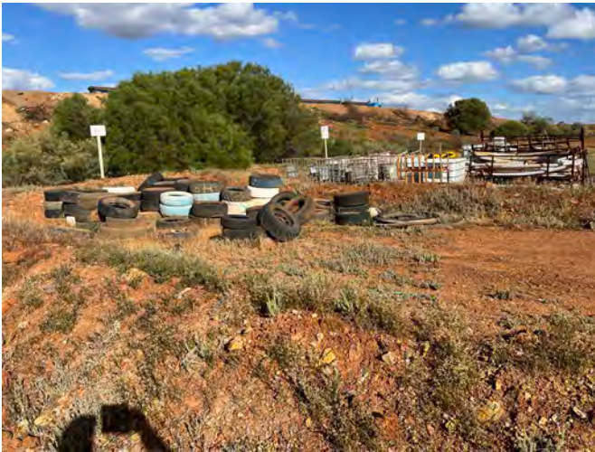
Figure 3-3: LV tyres in storage area - waiting burial in next tyre disposal cell (Oct 2025)
