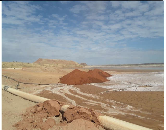
Plate 2 – Deposited material from toe drain in TSF Cell
