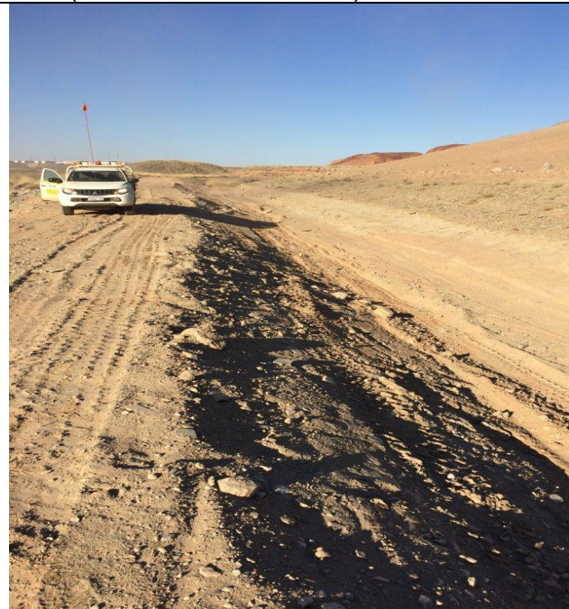
Plate 3 – Bund construction along and at end of toe drains – Eastern Wall
