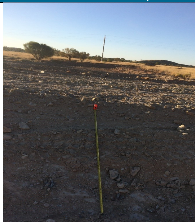
Plate 5 – Depth of construction of toe drain wall at location of erosion breach (sediment basin directly in front to provide water flow from surrounding environment).
