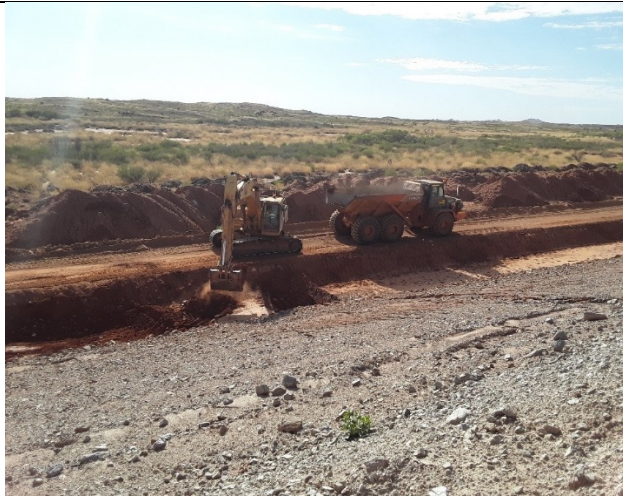
Plate 1 – Removal of Sediment from Toe Drains
