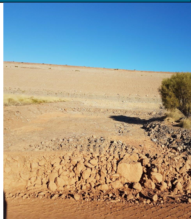
Plate 6 – Sediment basin constructed in front of toe drain (location of erosion breach) to remove excessive water flow away from toe drain infrastructure.
