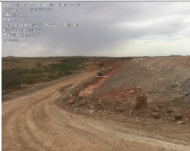
Plate 3 – Bund construction along and at end of toe drains – Eastern Wall
