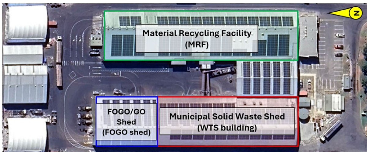
Figure 1: MRF, MSW shed and FOGO shed
