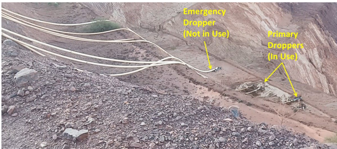
Figure I-3 View of Droppers from Near Manifold
