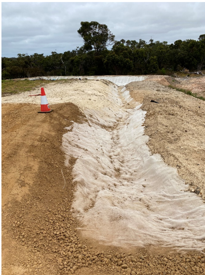
Figure 8: lined drainage channel
