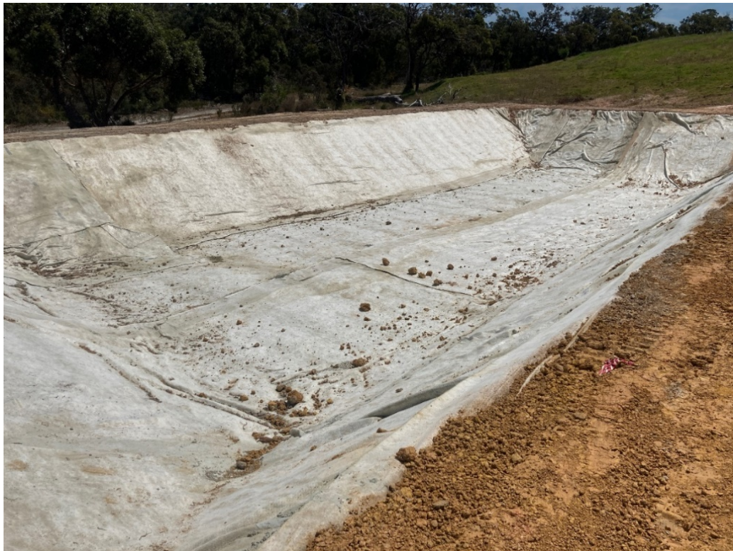
Figure 9: Lined leachate pond
