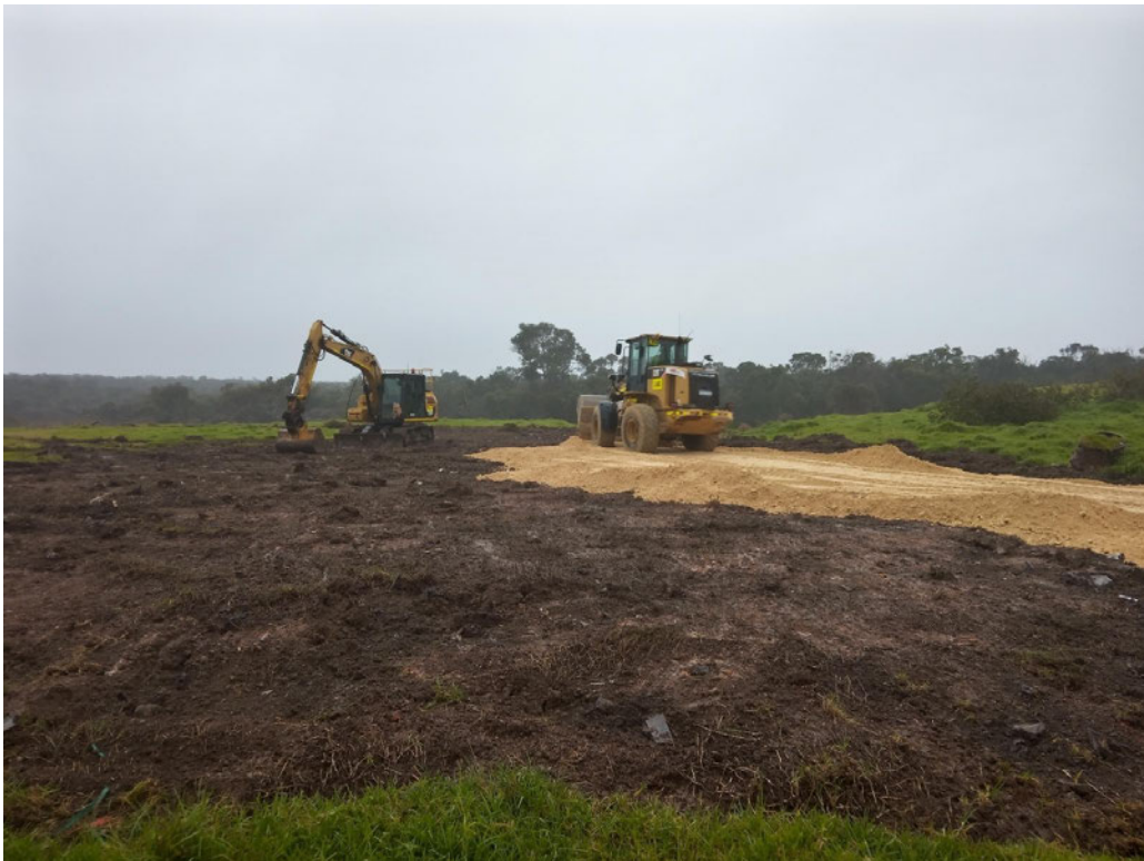
Figure 3: Top soil removal and laying of limestone sub base.
