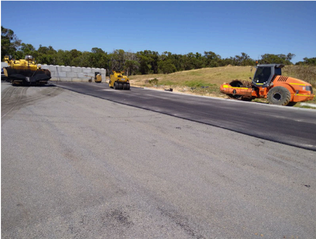
Figure 6: Partially sealed hardstand with Bund wall.
