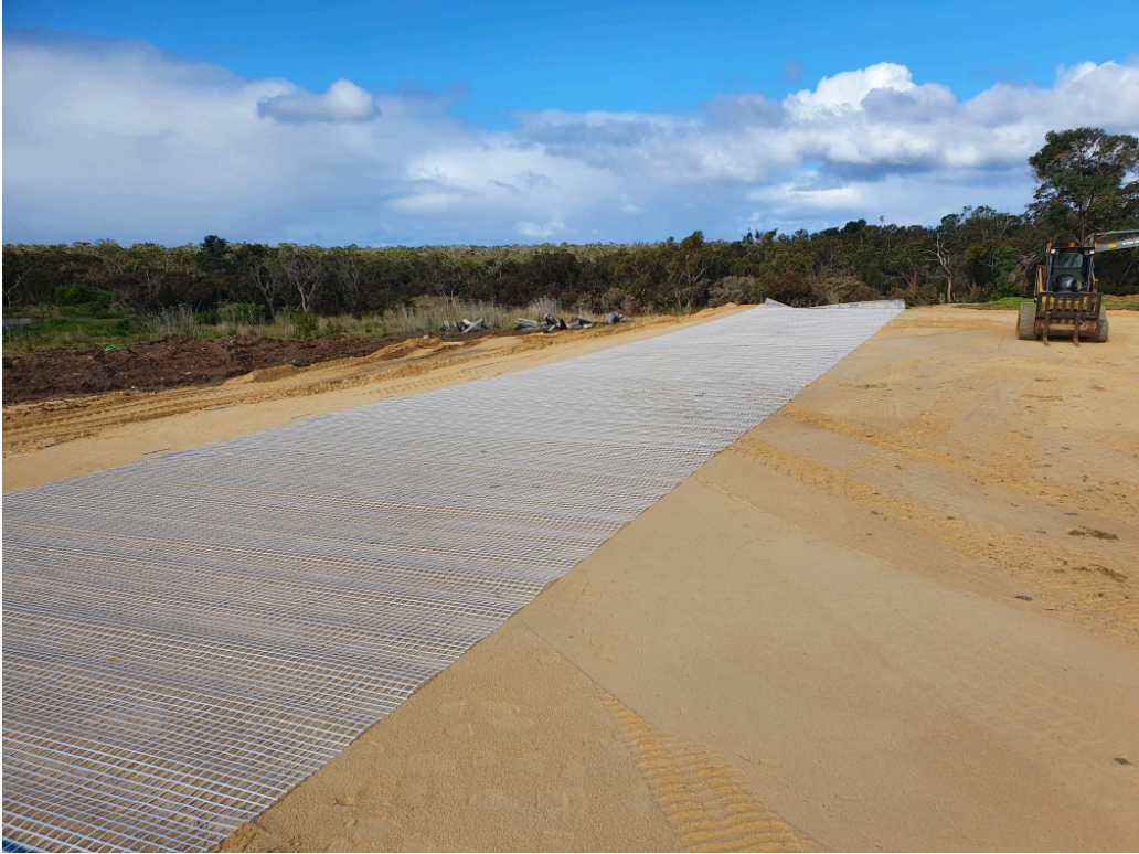
Figure 4: Installation of Geo Grid above limestone sub base.
