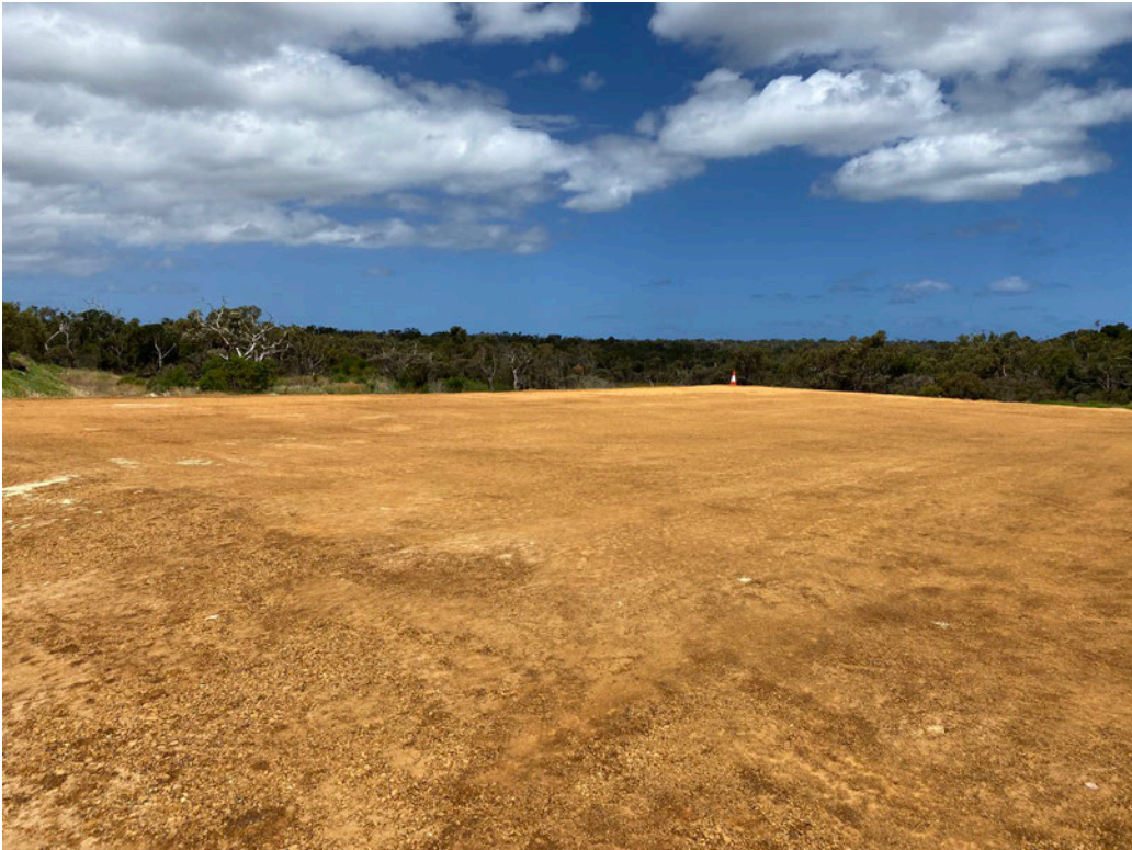
Figure 5: Prepared hardstand prior to sealing
