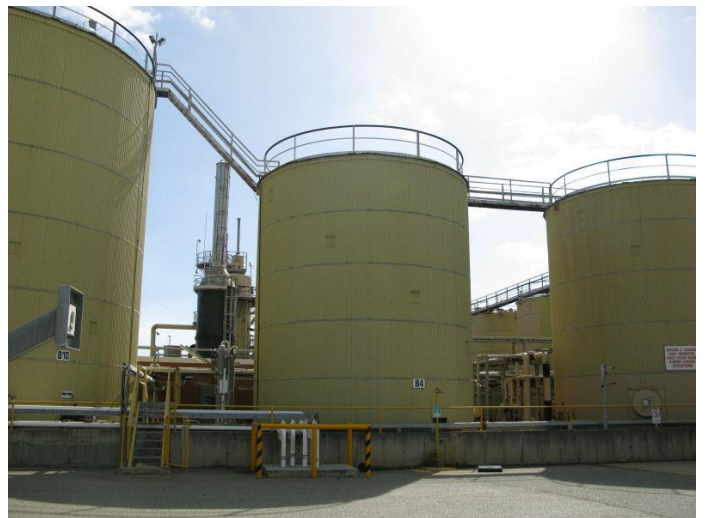
Bulk Fuel Terminal (DER, 2015)
