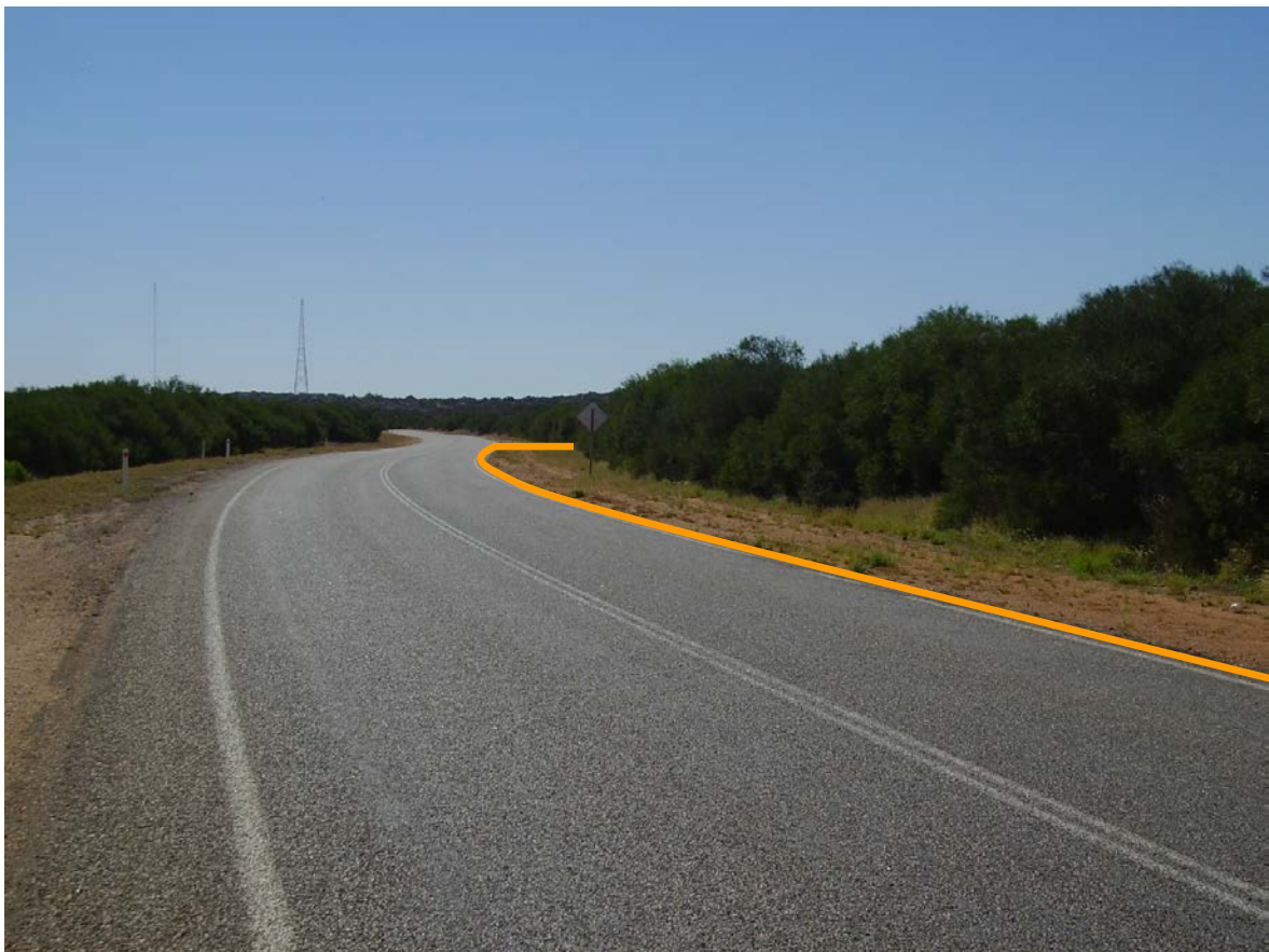
Photograph 8 – Six Mile Creek Side Access Track (467.78 SLK) North View
