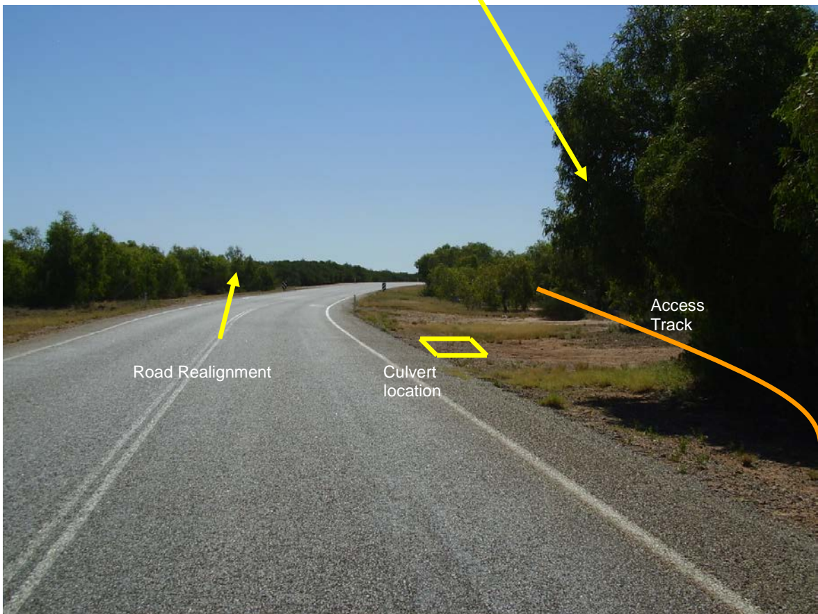
Photograph 2 - Six Mile Realignment (467.65 SLK) North View
