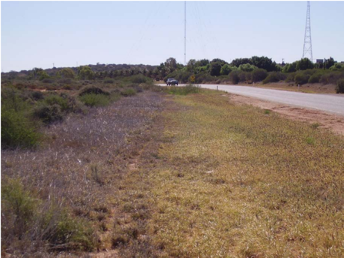
Photograph 5 – Northern End of Proposed Six Mile Realignment (469.07 SLK) North View
