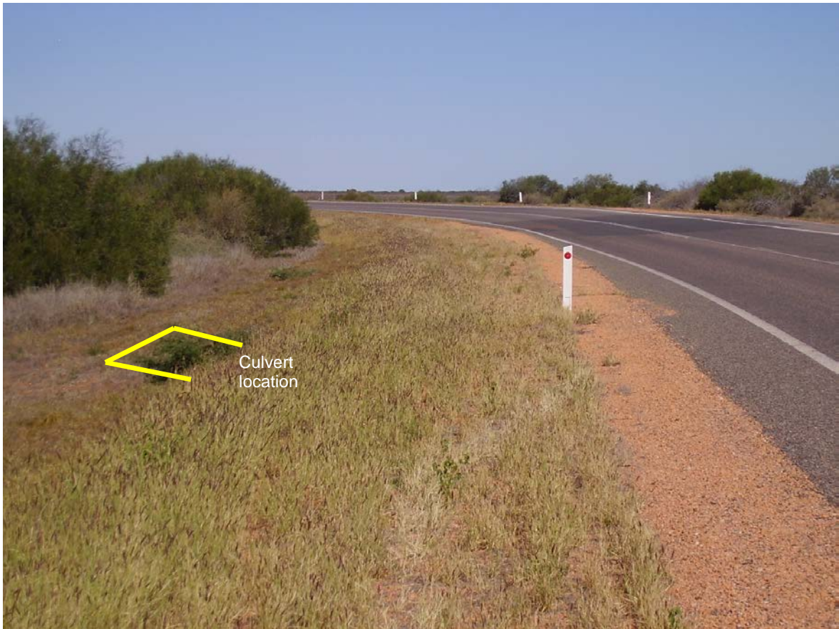
Photograph 10 – Drag Strip Culvert Upgrade Location (462.8 SLK) North View
