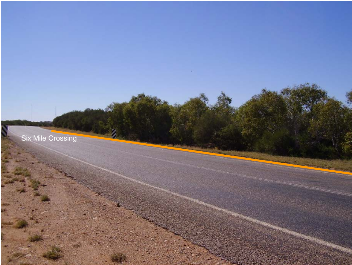
Photograph 7 – Six Mile Creek Side Access Track (467.65 SLK) North View
