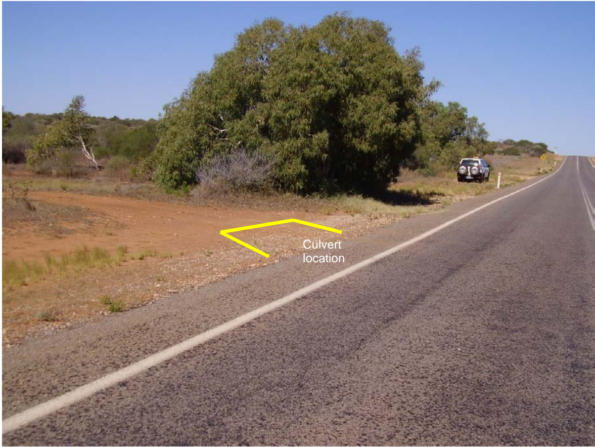
Photograph 9 – Six Mile Creek Culvert Relocation (467.55 SLK) North View
