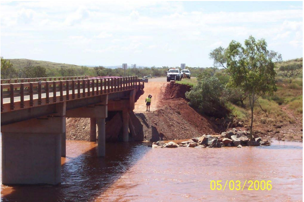
Photograph 2. Duck Creek Flood Damage - Nanutarra Munjina Rd - 62.29 SLK- North West View
