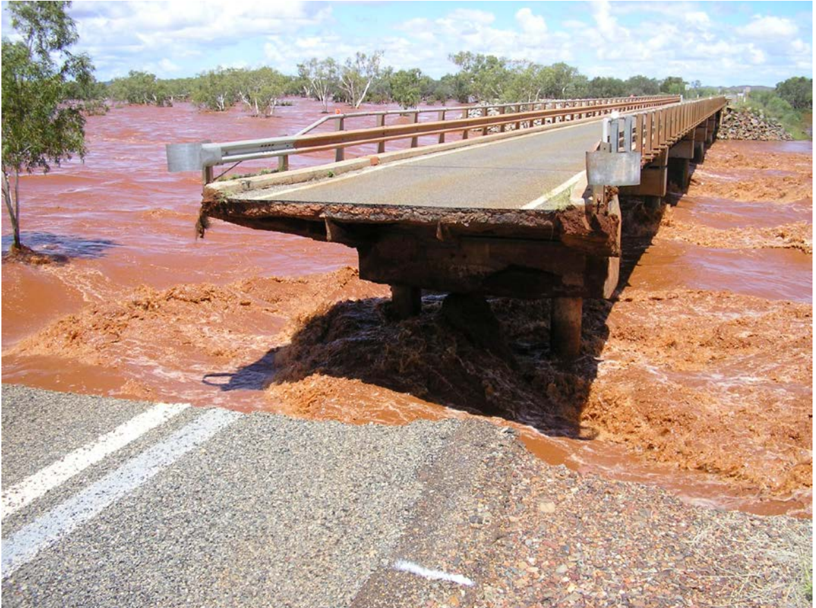
Photograph 1. Duck Creek Flood Damage - Nanutarra Munjina Rd - 62.29 SLK- South East View
