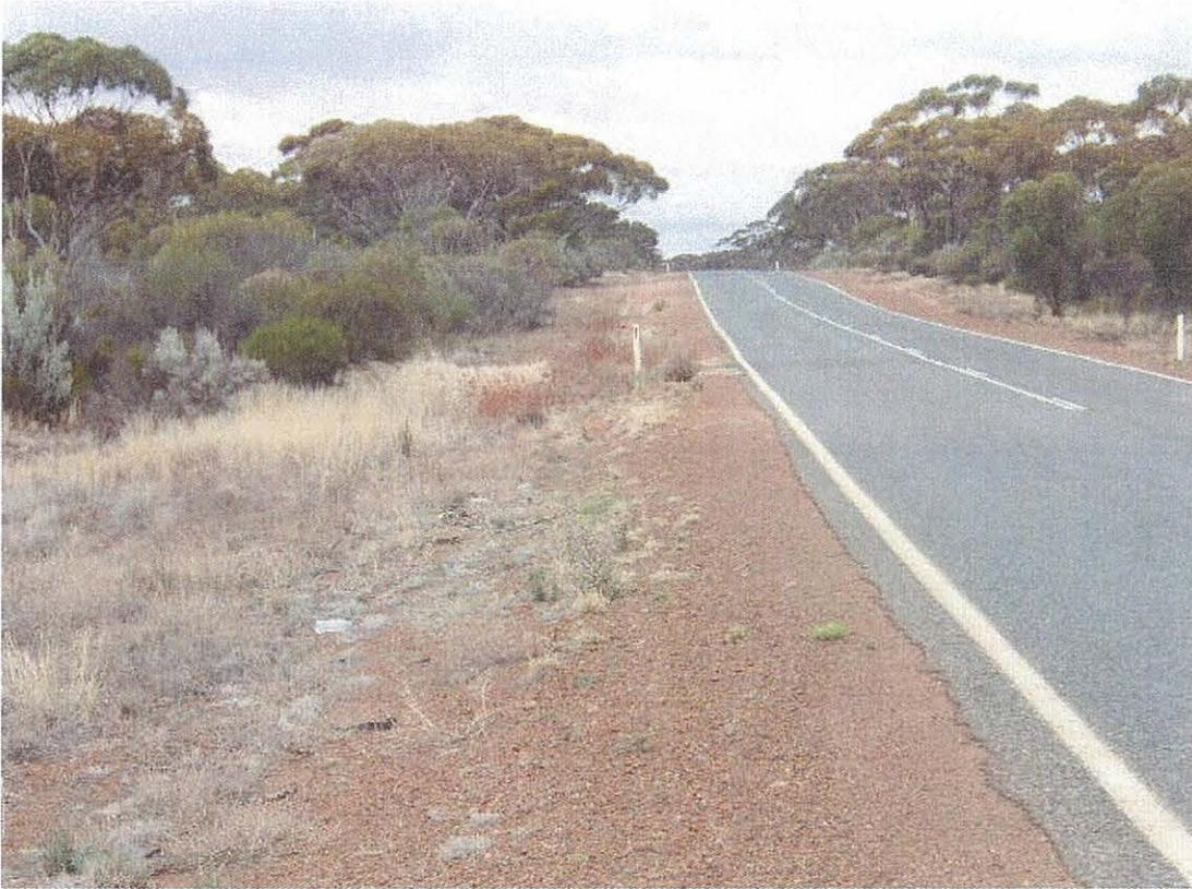
Guide Post indicates approximate position of the edge of the new formation. Note grass on edge of roadway will need to be cleared.
