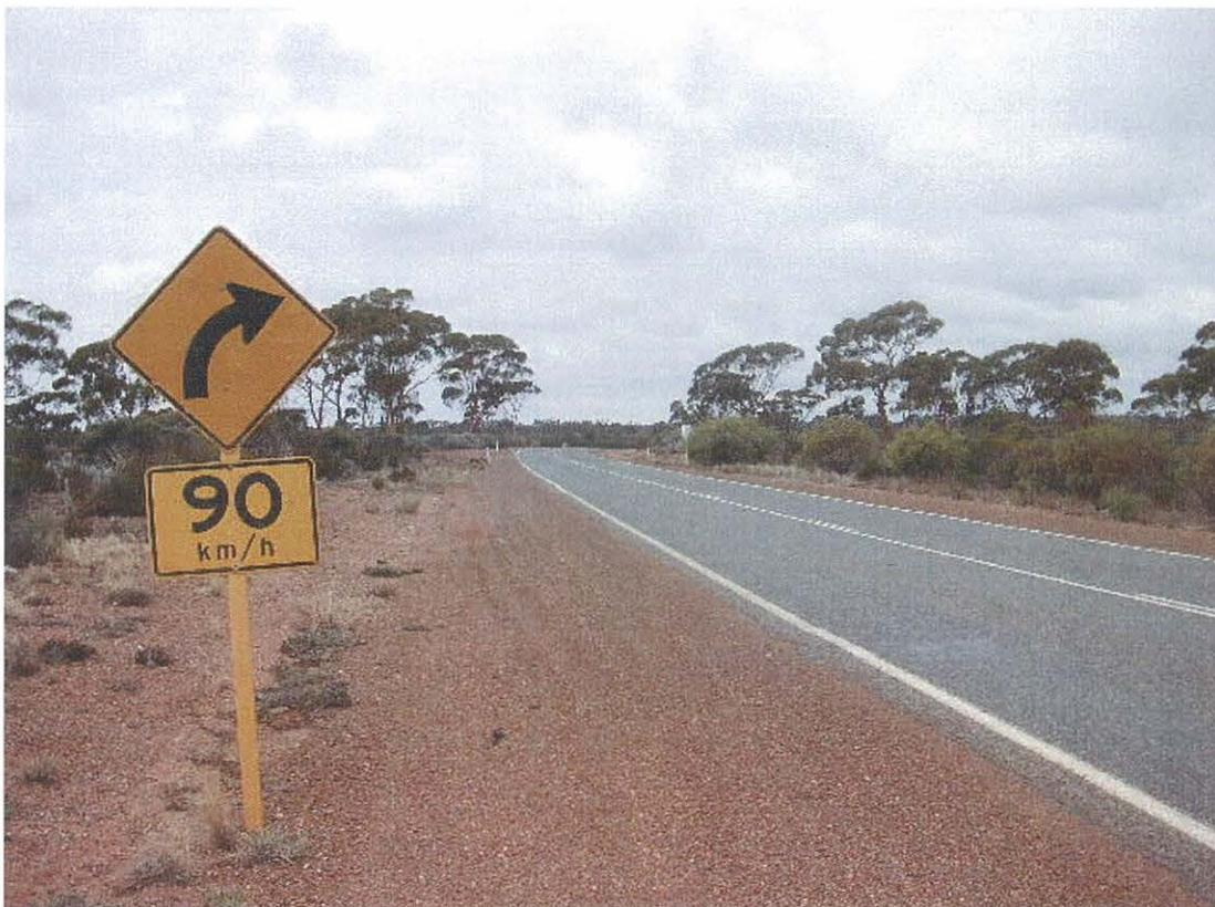
Possible realignment (minor) required on this curve to improve horizontal geometry
