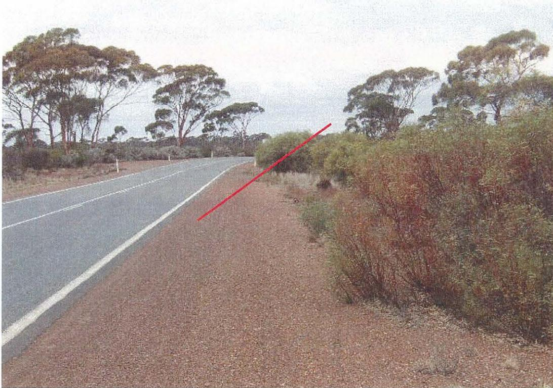
Possible realignment required on inside of curve to improve horizontal geometry. Red line indicates approximate area required for realignment.
