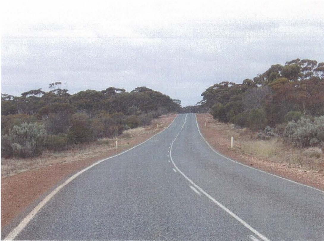
Photo Emu Rocks to Widgiemooltha Project looking south along the Great Eastern Highway. Existing seal width approximately 7m. Planned seal width 8m on 10m wide formation. Guide Post shown in photo are approx 9.8m
