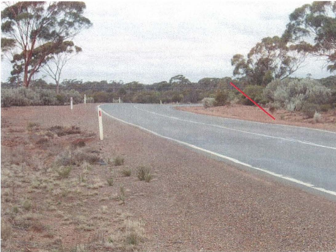
View of vegetation on inside of curve that may need to be cleared to facilitate improvements in the horizontal geometry.
