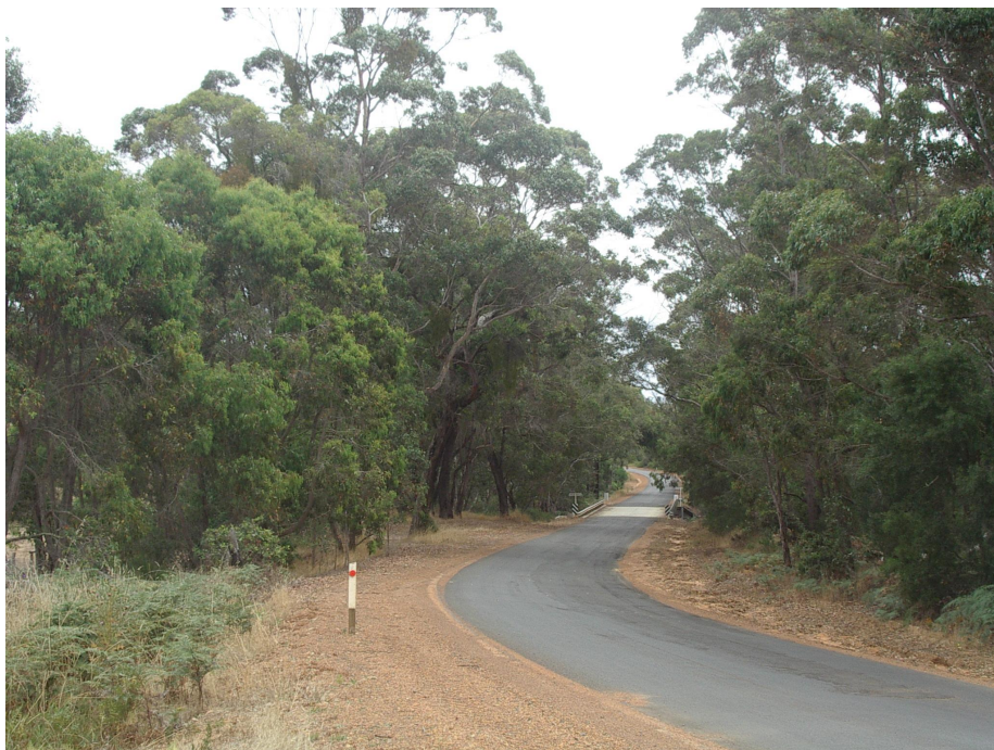
Photo 4: Eastern approach to Perup River bridge looking west
