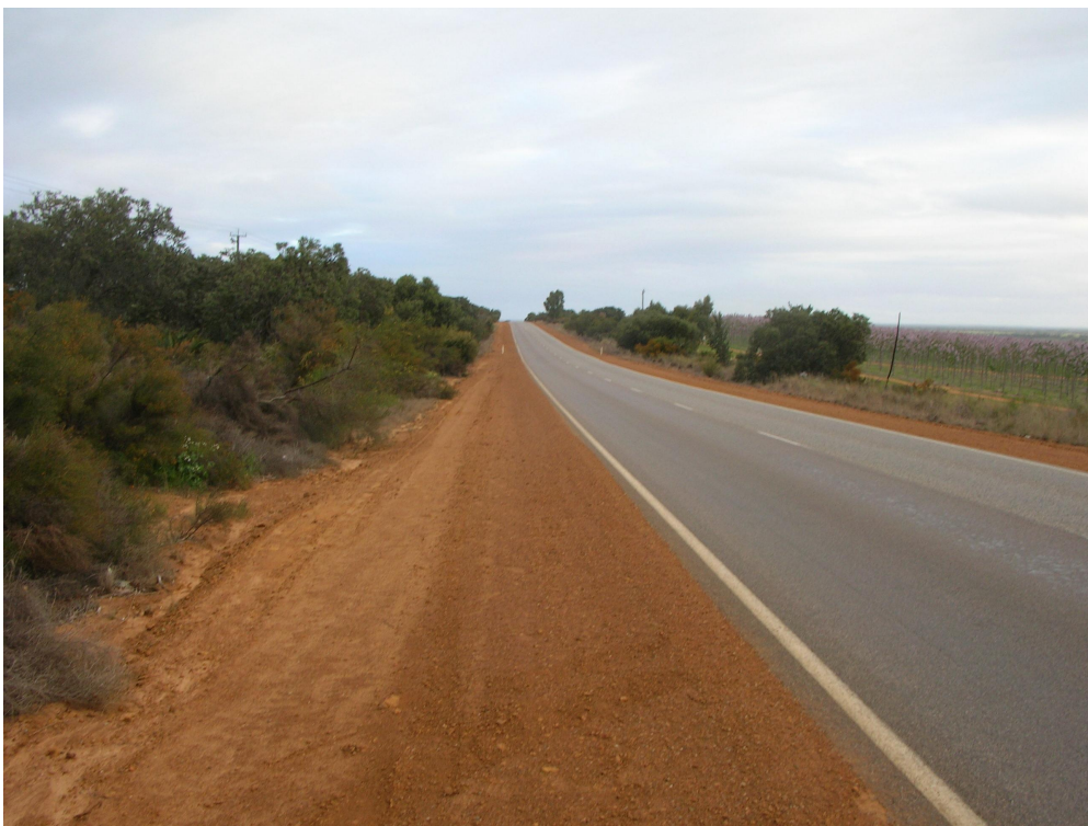
Plate 3: Northern section of site shows degraded road reserve on the west side of the highway, with native vegetation in better condition on east of highway. Photo taken looking south.
