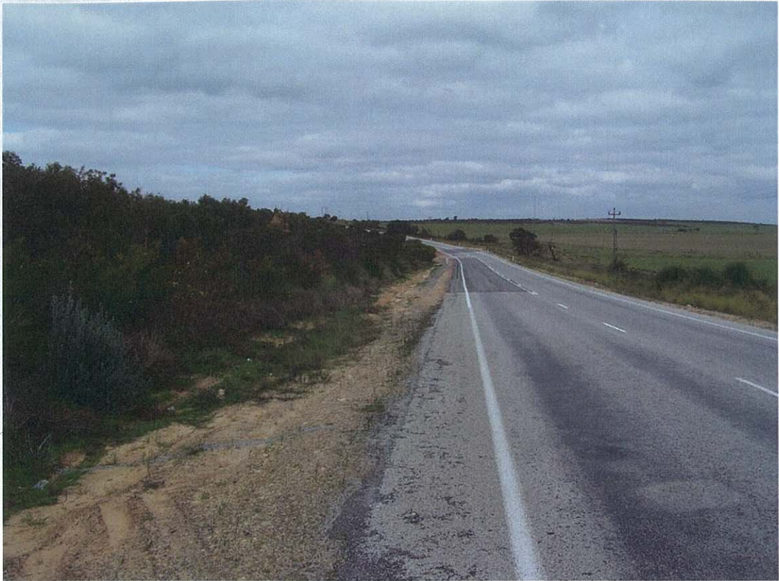
37.5 SLK, (Right Hand Side) - facing South
