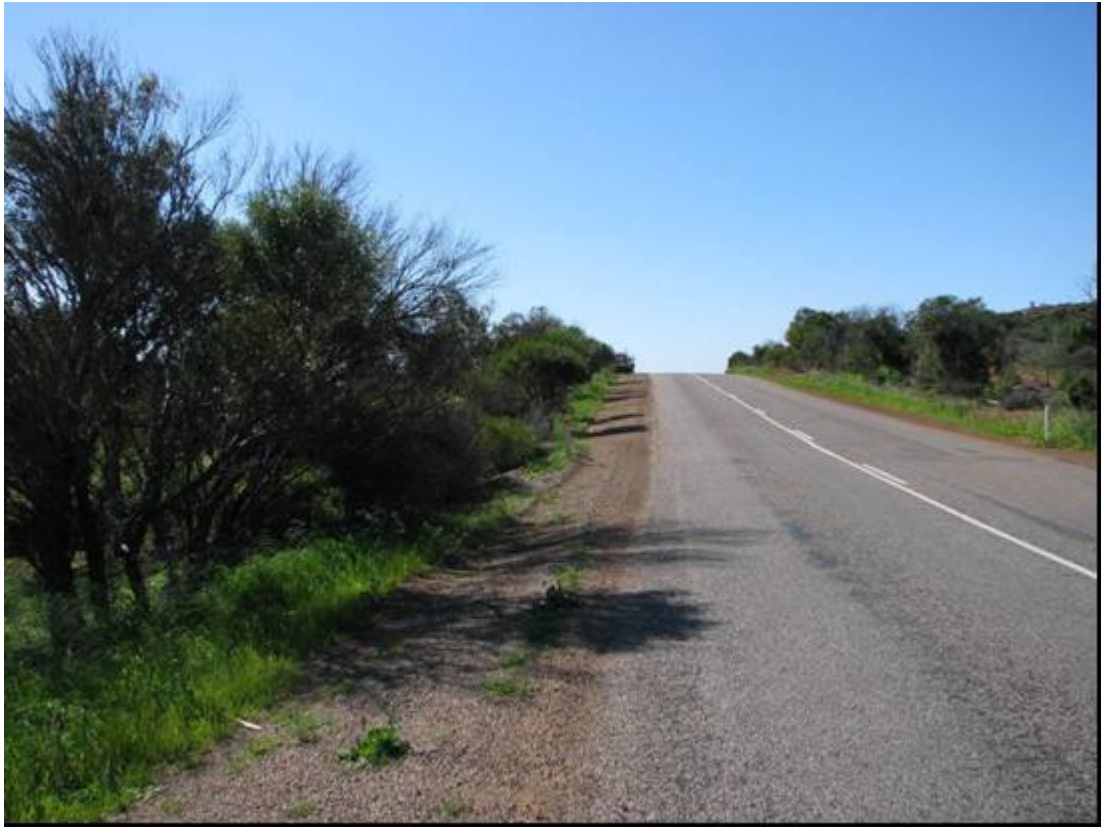
Figure 1: Photo facing north along the west side of the road
