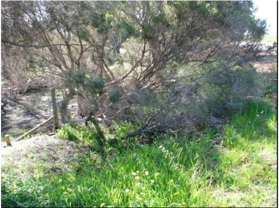
Figure 9: Photo of culvert that requires cleaning/clearing out
