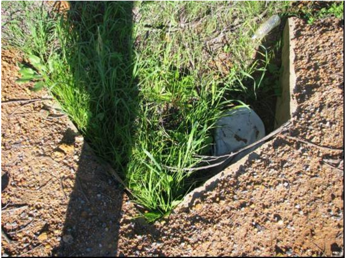
Figure 19: Photo of culvert that requires cleaning/clearing out
