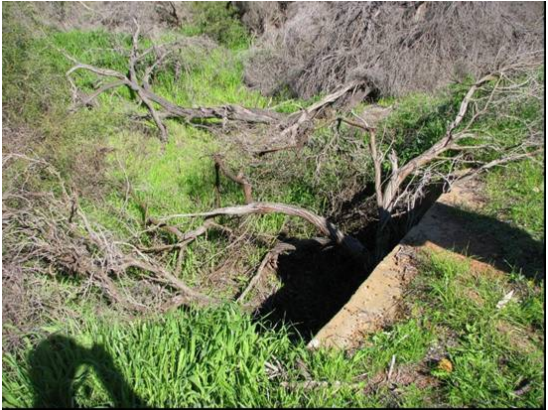
Figure 13: Photo of culvert that requires cleaning/clearing out
