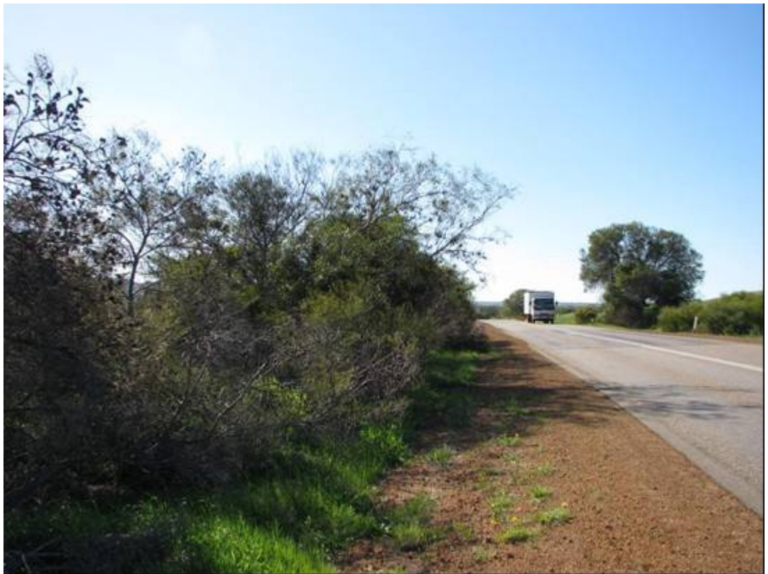
Figure 10: Photo facing north along the west side of the road
