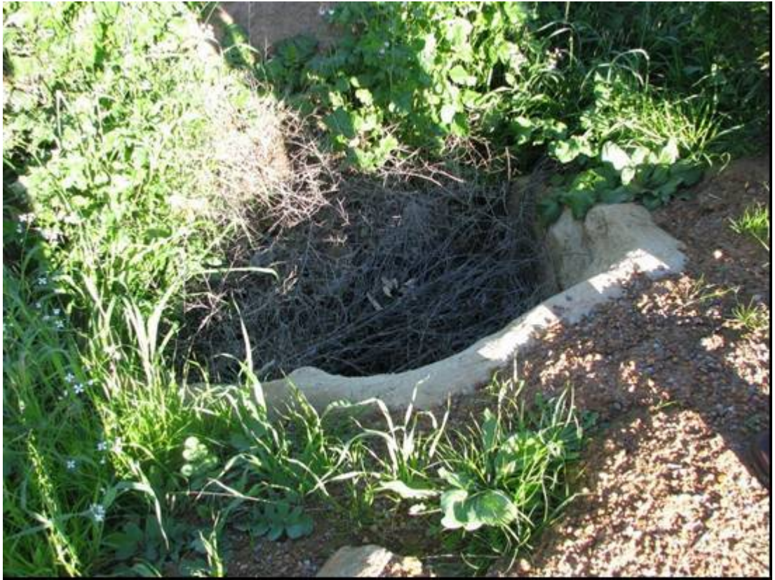
Figure 17: Photo of culvert that requires cleaning/clearing out
