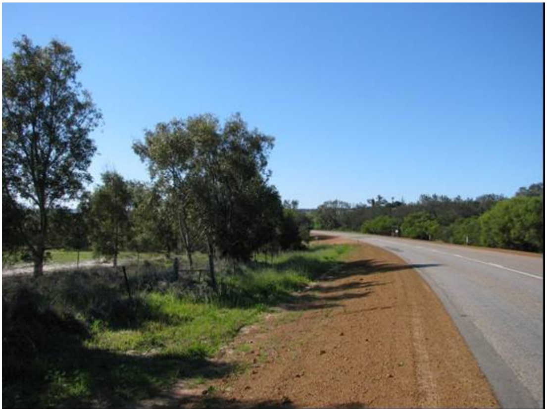
Figure 8: Photo facing north along the west side of the road.
