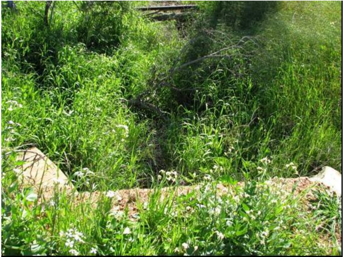
Figure 7: photo of culvert that requires cleaning/clearing out
