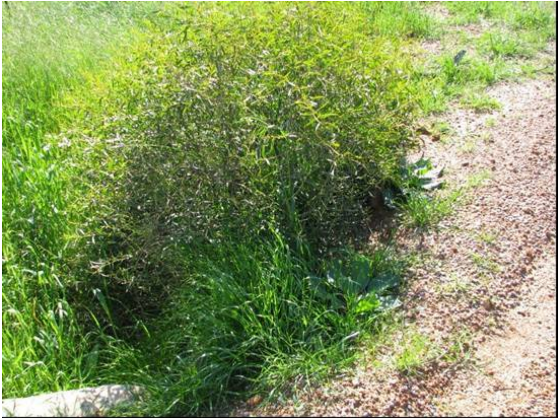
Figure 3: Photo of culvert that requires cleaning/clearing out
