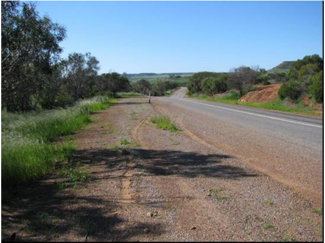
Figure 5: Photo facing north along the west side of the road
