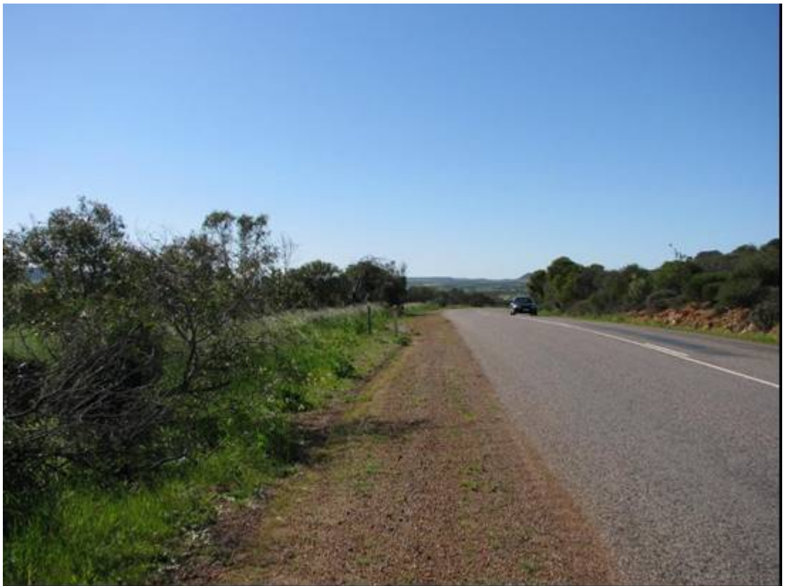
Figure 2: Photo facing north along the west side of the road
