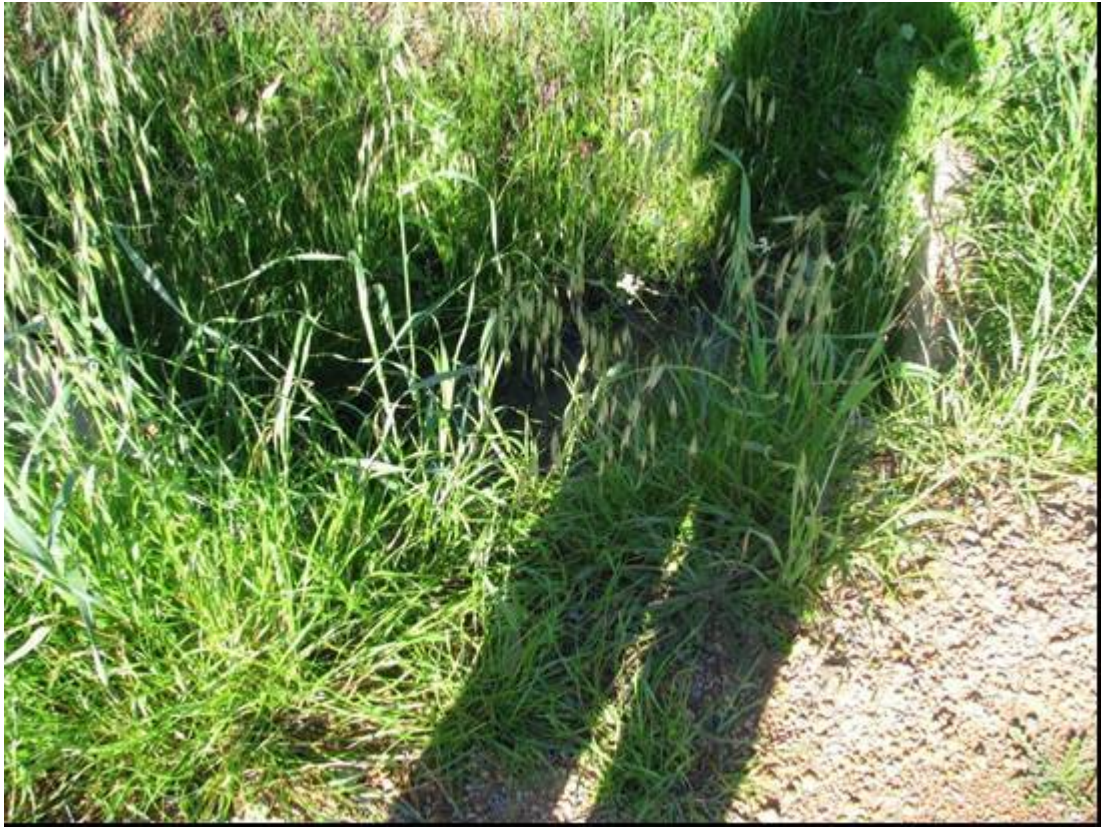
Figure 21: Photo of culvert that requires cleaning/clearing out
