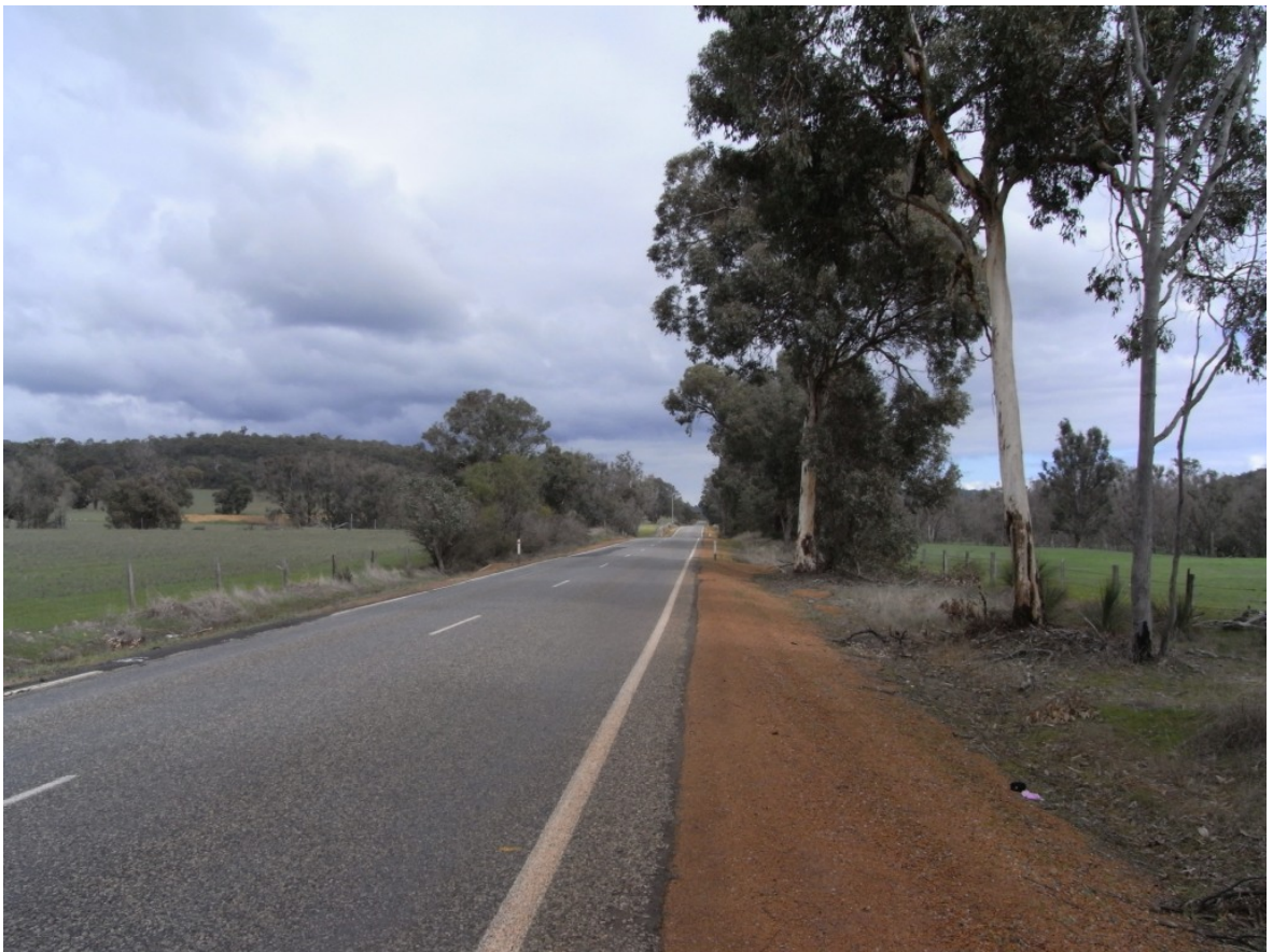
Photo 1: View south – clearing to be undertaken on the left side of the road
