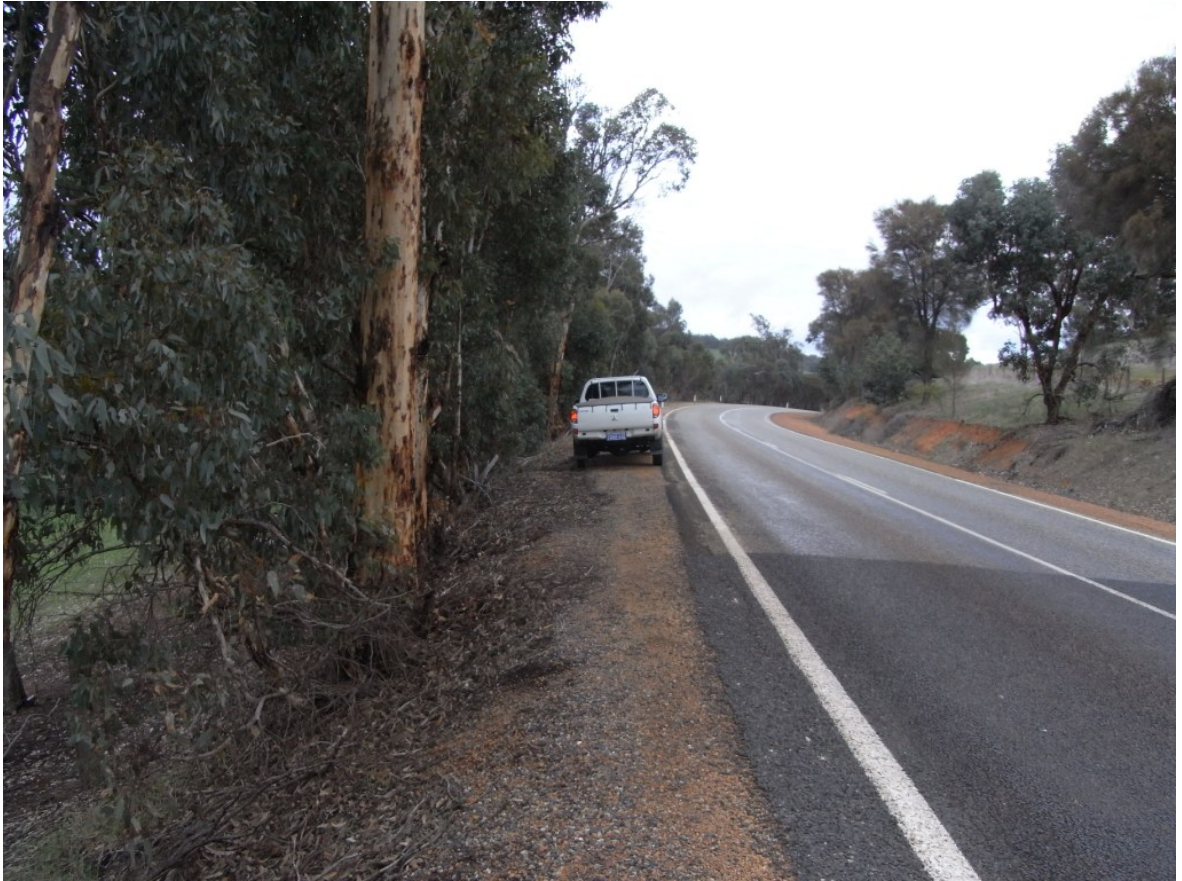
Photo 4: View north - clearing to be undertaken on the right side of the road with individual trees removed from the left
