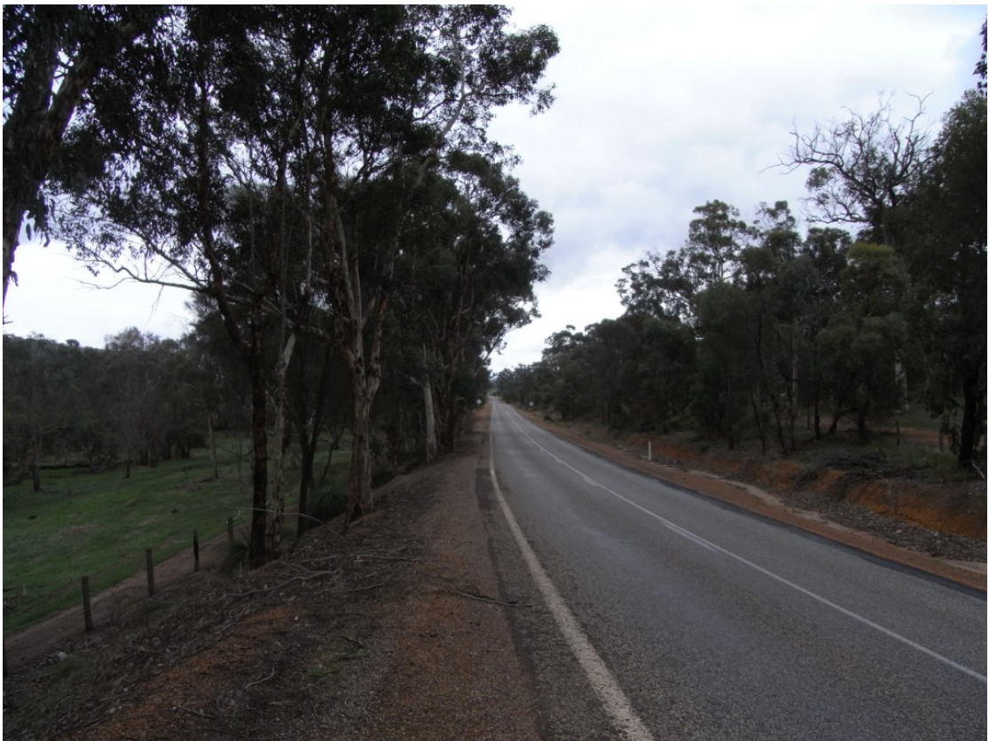
Photo 3: View north - clearing to be undertaken on the right side of the road with individual trees removed from the left
