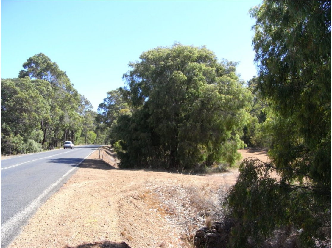
Photo 2: View north - clearing to be undertaken on the right side of the road. Note width of vegetation between the highway and the state forest track. Also note the drop-off within metres of the road edge.
