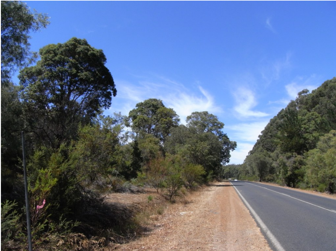
Photo 7: view south showing vegetation on the left to be removed
