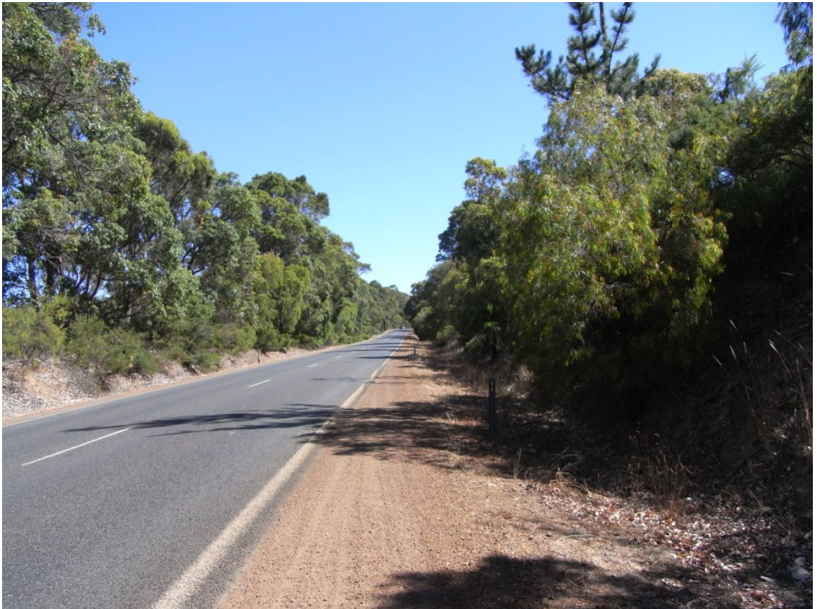
Photo 1: View north at SLK 94 – clearing to be undertaken on the right side of the road
