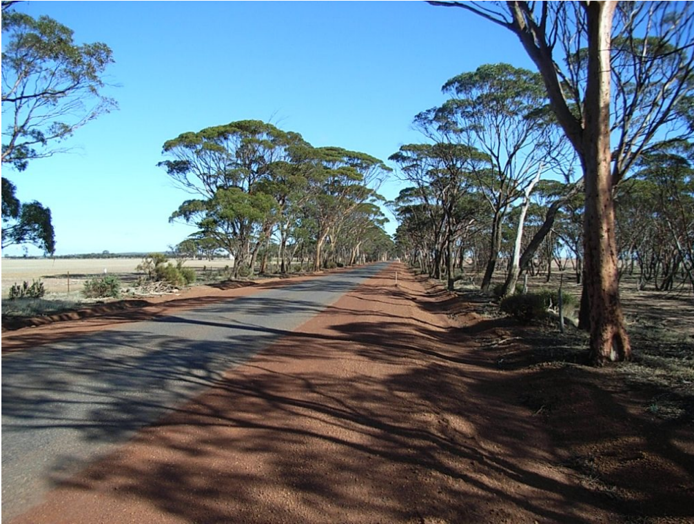
View west SLK 232.8 (Note vegetation in paddock outside of proposed clearing area)
