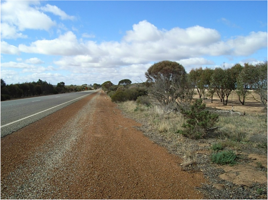
View east SLK 235.1 (Note established revegetation on the right)
