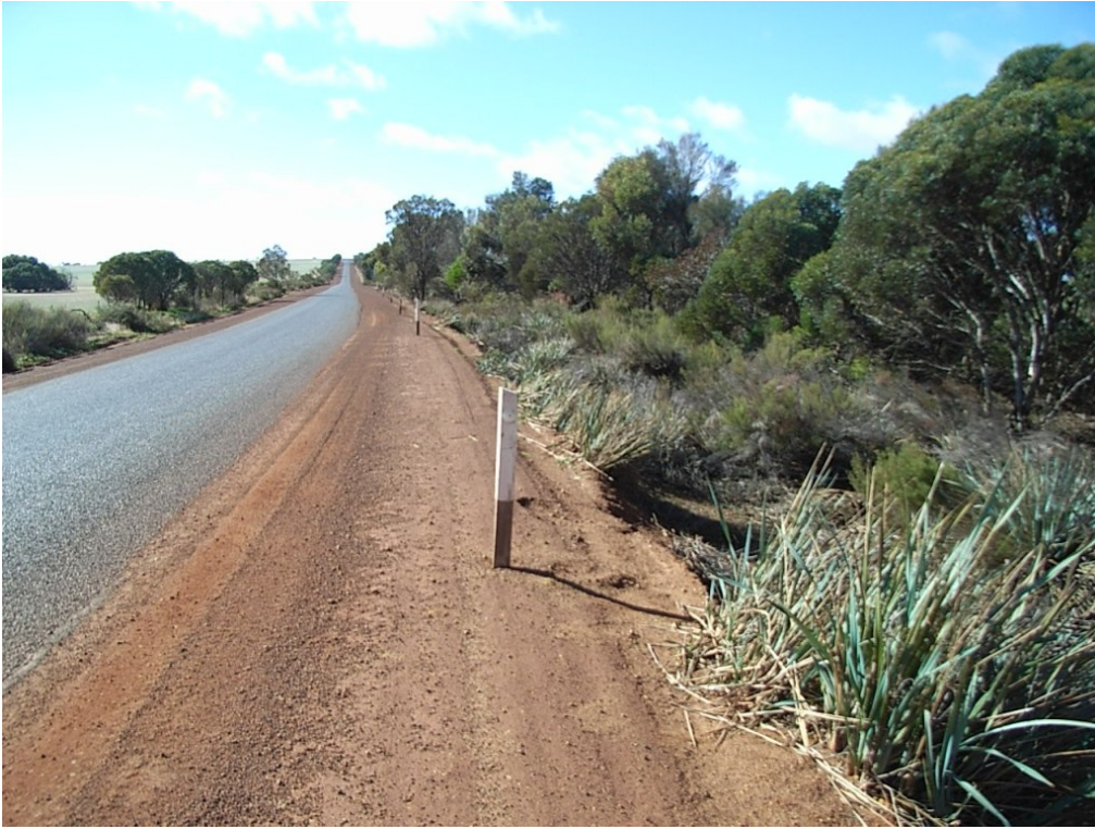
View east SLK 233.6 (Note established revegetation on the right)
