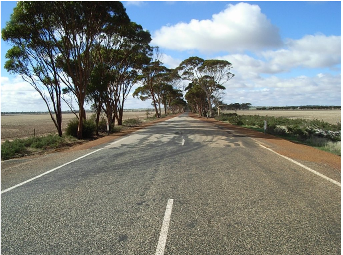
View east SLK 231.3: western end of project (Note the transition from two to single sealed lanes)
