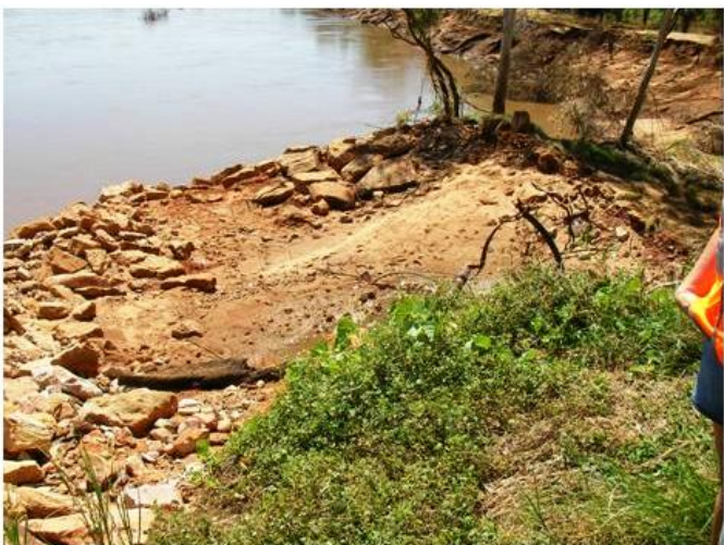
Remaining Abut 2 LHS Guidebank After to Flooding
