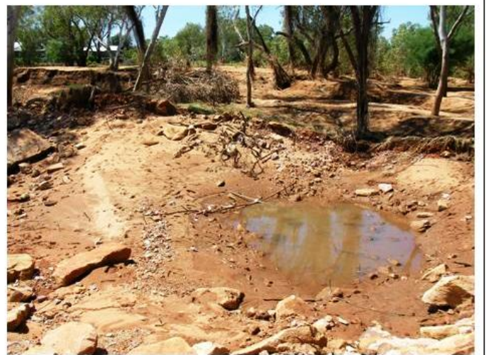
Remaining Abut 2 LHS Guidebank After to Flooding with Silt Deposits Behind Guidebank
