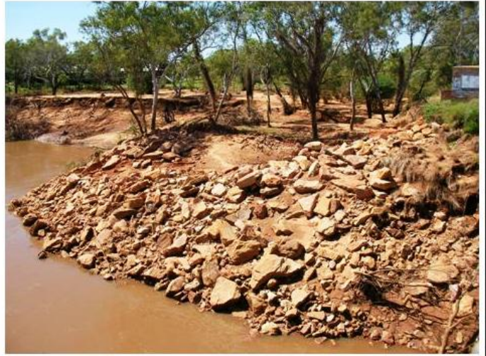
Abutment 2 LHS Guidebank After to Flooding
