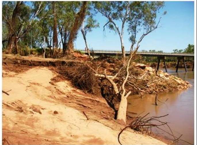
Abutment 2 LHS Guidebank After Flooding
