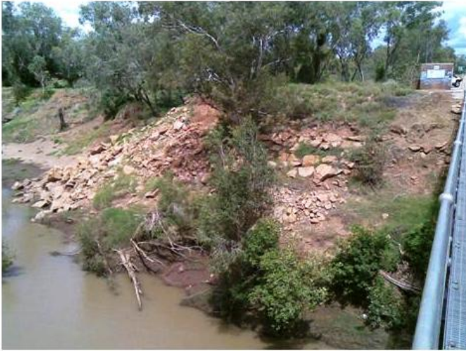
Abutment 2 LHS Guidebank Prior to Flooding current original
