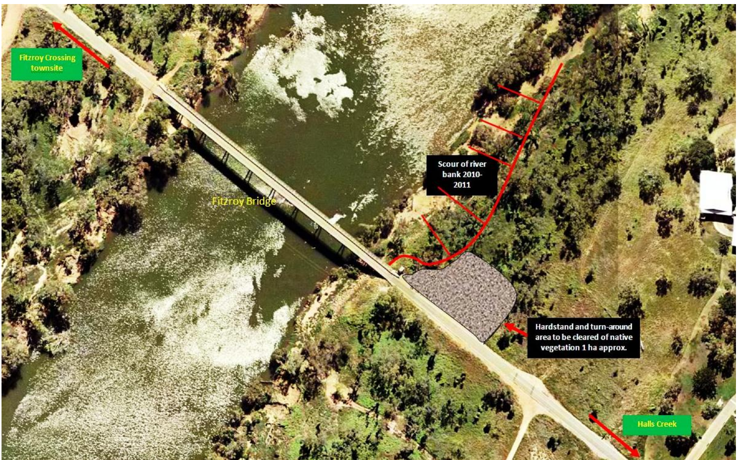
Figure 2...Close-up image of project area and location of clearing activities.
