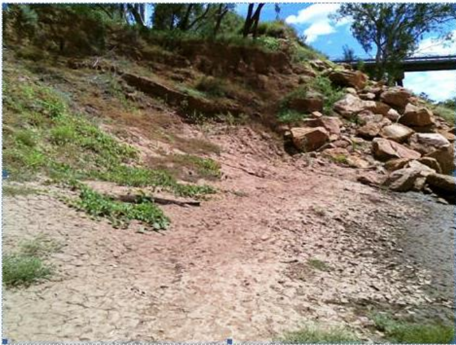
Abutment 2 LHS Guidebank Prior to Flooding
