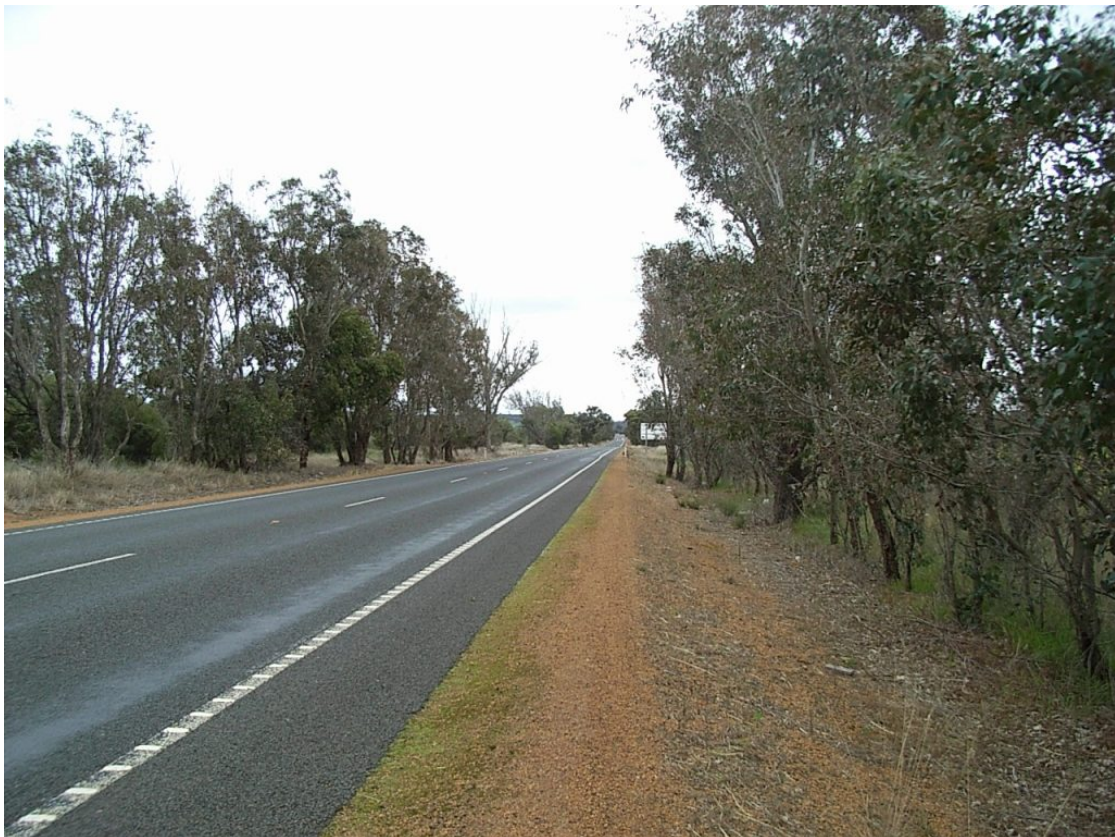
Photo 3: SLK 144.86 - Shows a 5m clear zone in the foreground and 3.5m in the background
