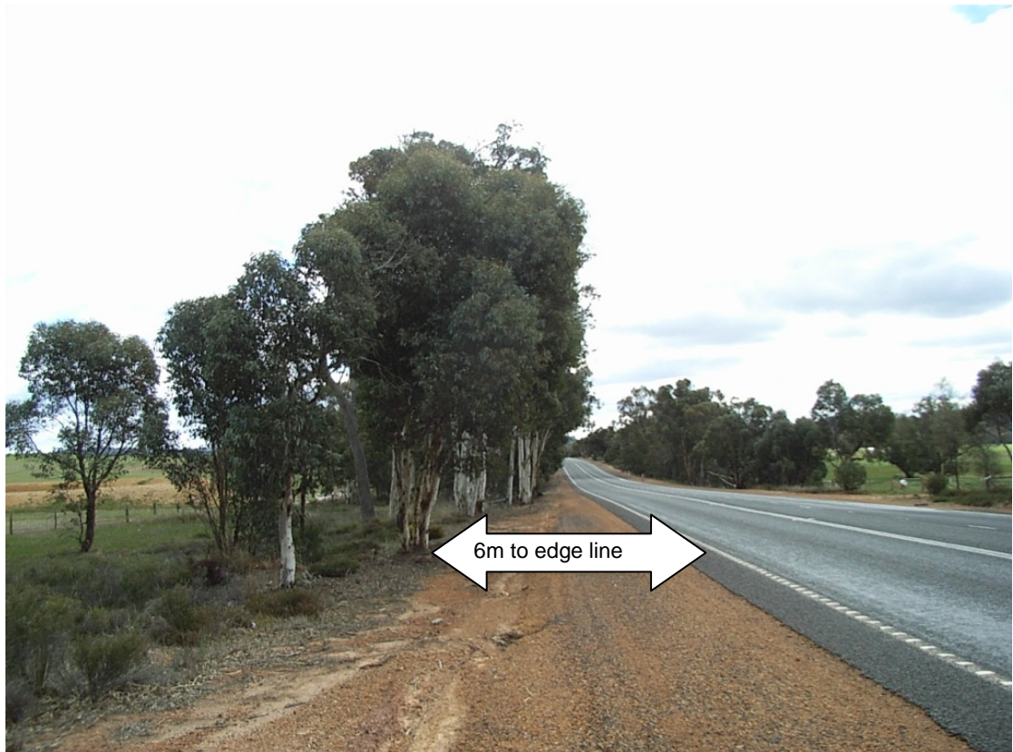
Photo 1: SLK 136.83 - Indicates the proposed clear zone width for straight sections of road
