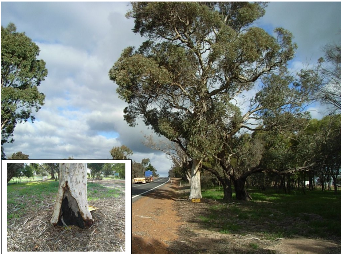
Photo 9: SLK 165.67 – Large tree 3.5m from edge line with hollow base (inset photo)
