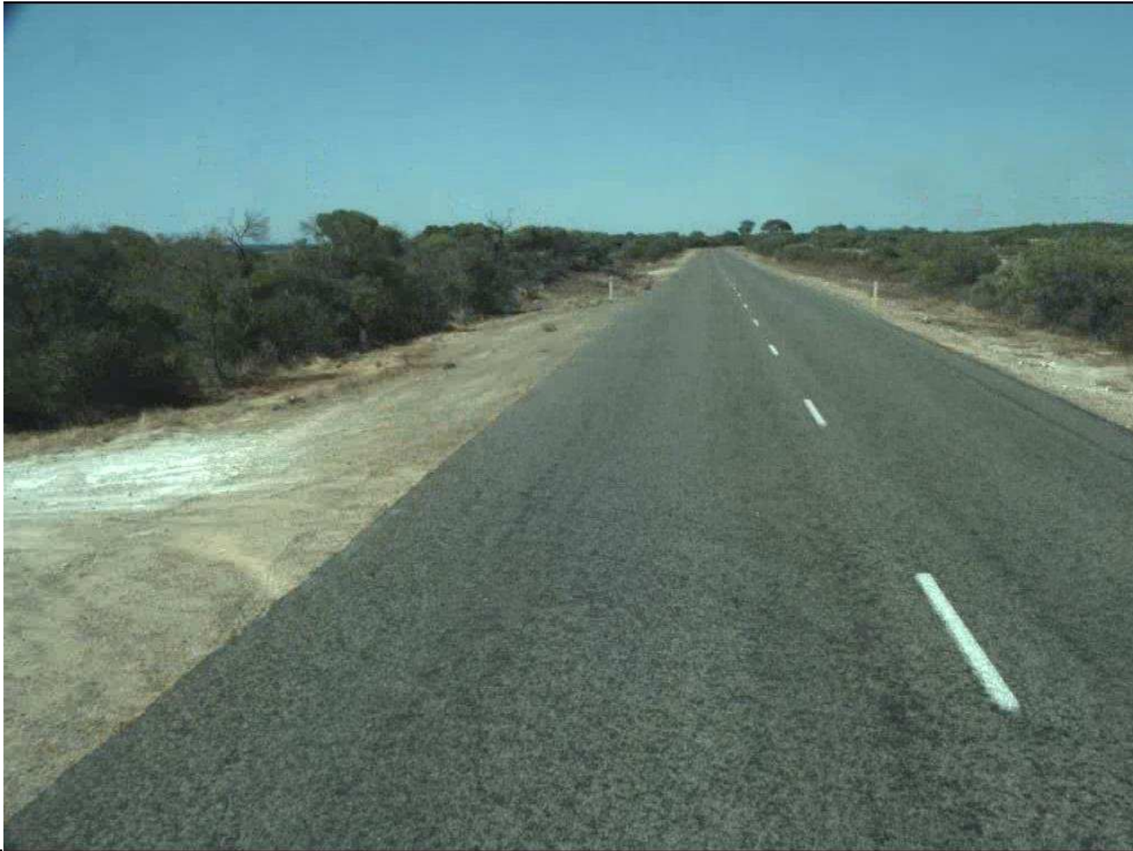
Photo 2: Looking North Taken 19/01/2010 at SLK 246.6
