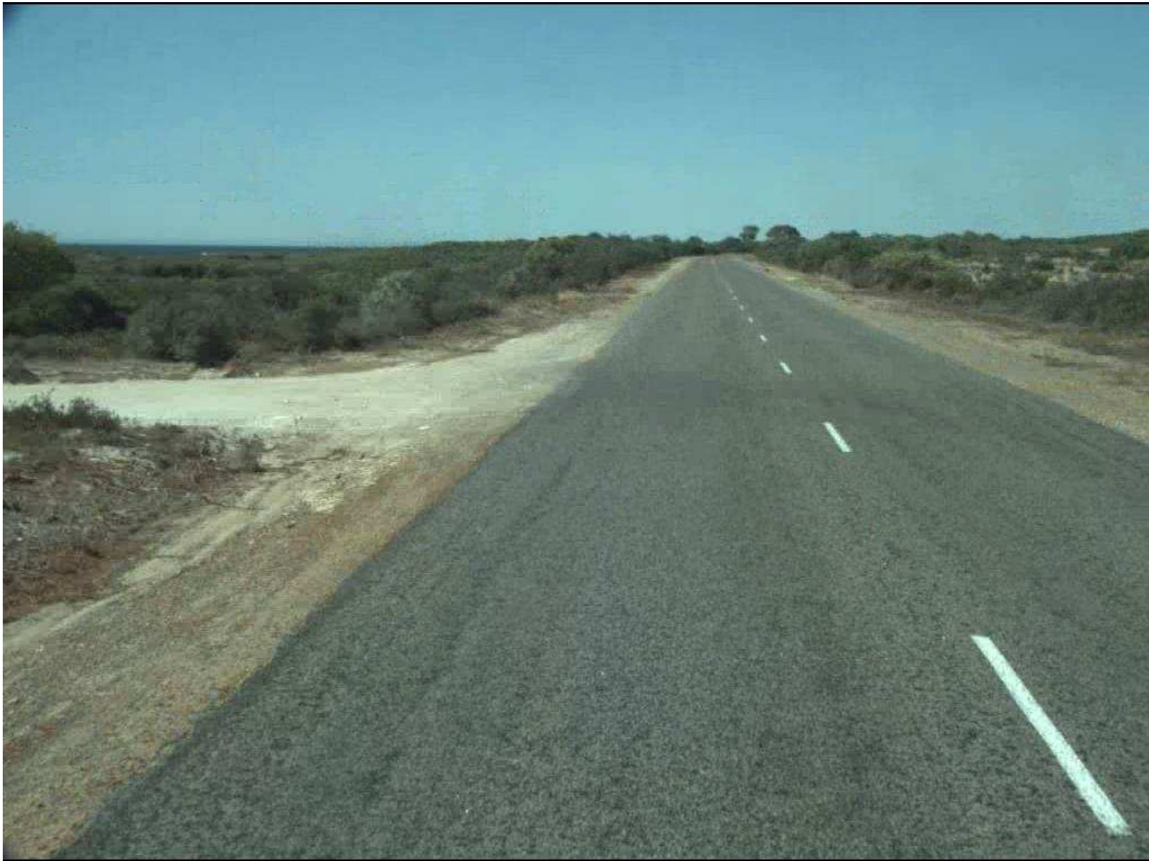
Photo 3: Looking North Taken 19/01/2010 at SLK 246.
