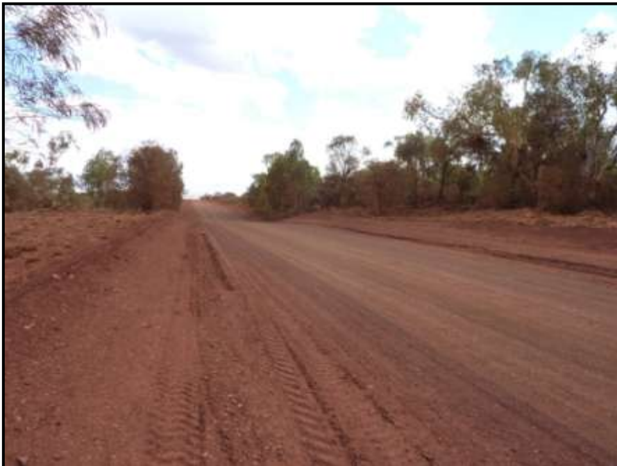
Photo 2: M030 Kalgan floodway facing south
