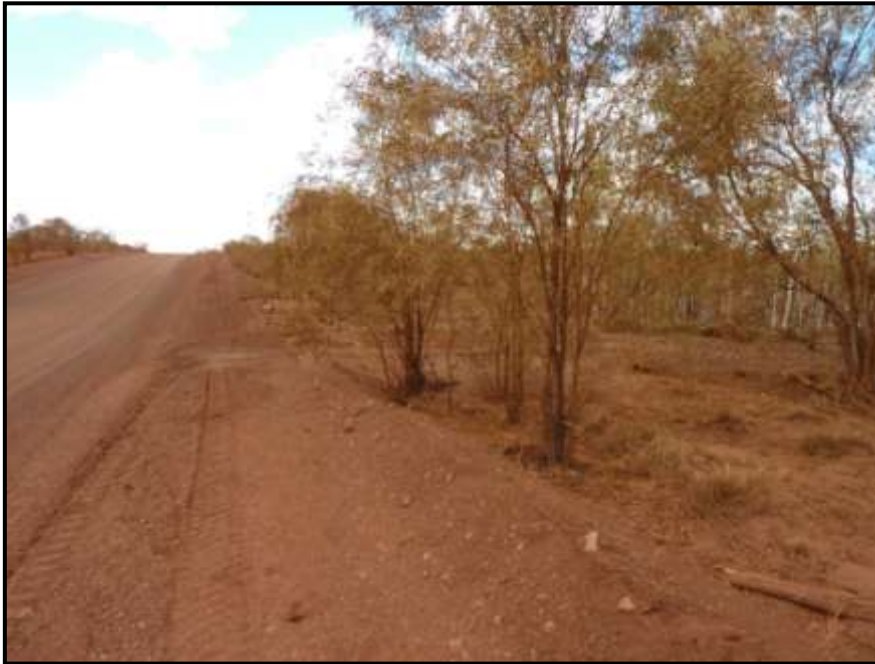
Photo 1: M030 Kalgan floodway facing north
