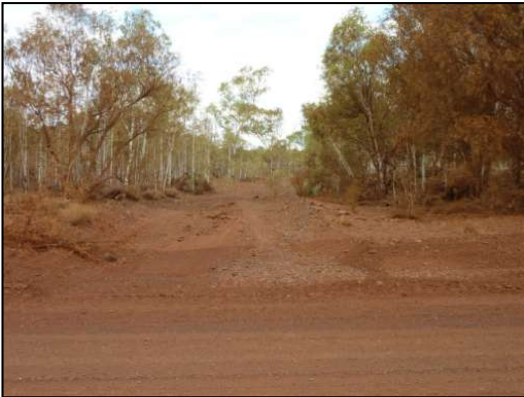
Photo 4: M030 Kalgan floodway side track
