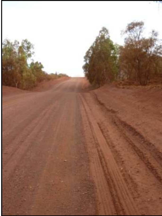
Photo 5: M030 Kalgan floodway facing south
