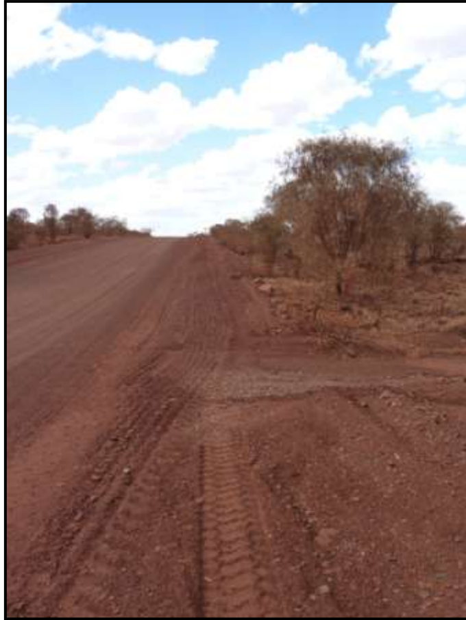
Photo 3: M030 Kalgan floodway facing north
