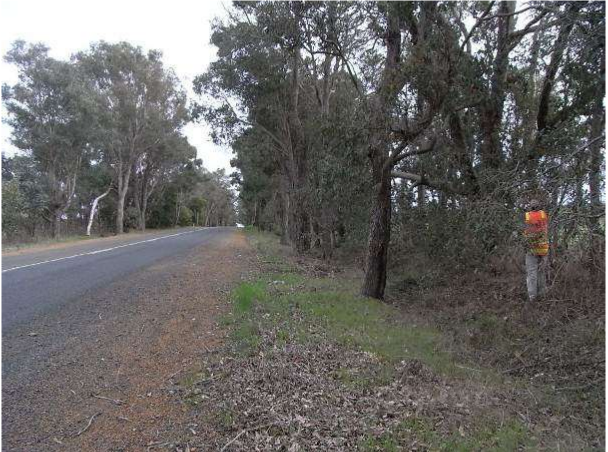
Photo 5: View west from SLK 118.25 showing trees in the table drain
